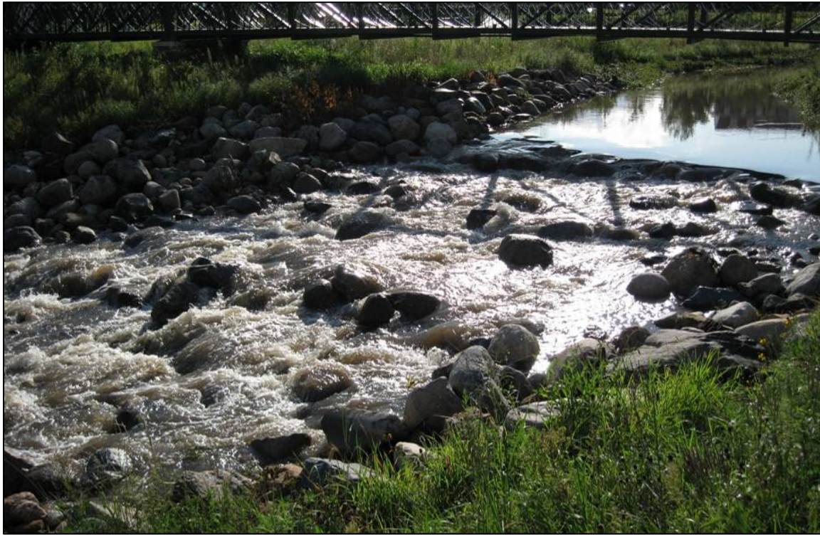
Figure 2.3 Rock Cascade #2 at Reach 7 at high flow.
