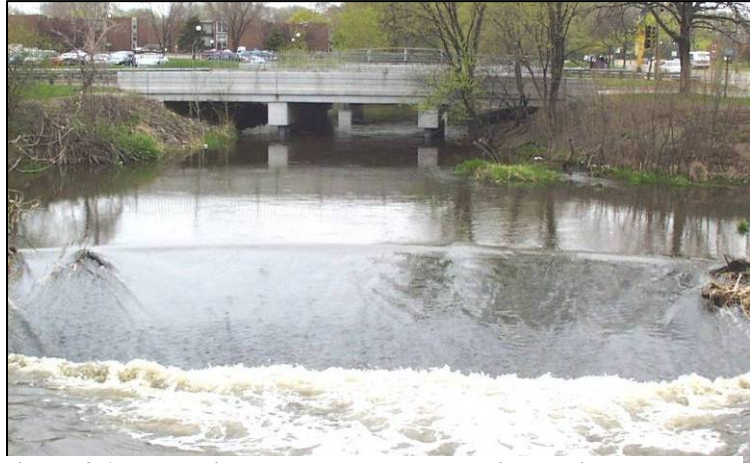
Figure 2.1. Reach 4, the Bass Lake Road weir, looking upstream.
