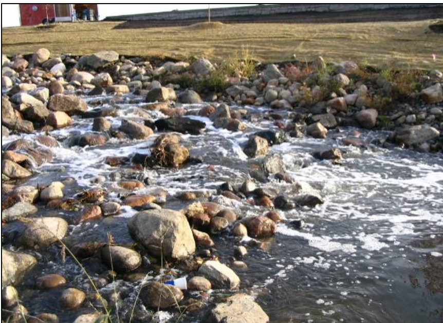
Figure 2.2. Rock Cascade #2 at Reach 7 at low flow.
