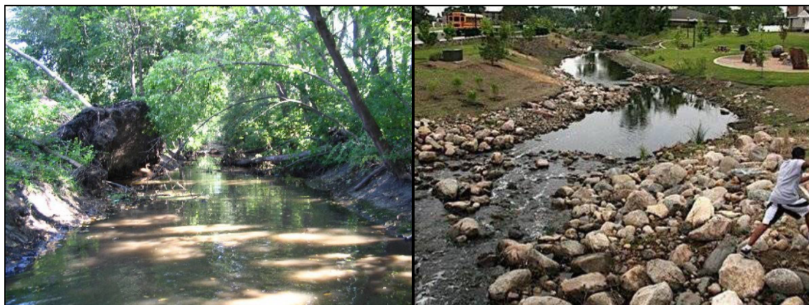
Figure 4.16. Reach 8 before reconstruction (left) and after (right).
