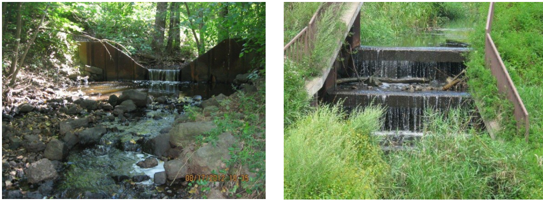
Figure 4.24 Examples of drop structures and step-weir structures along Battle Creek.
