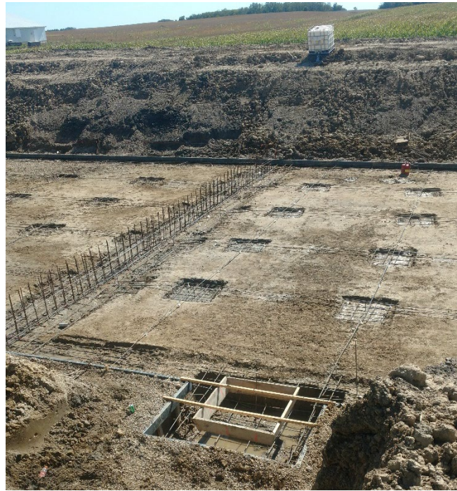
Liquid manure storage area under construction
