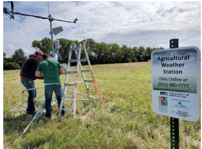
Figure 32. Dakota County SWCD and MDA staff installing an ag weather station. Access to current weather is critical for growers to efficiently schedule irrigation and reduce nitrate leaching.
