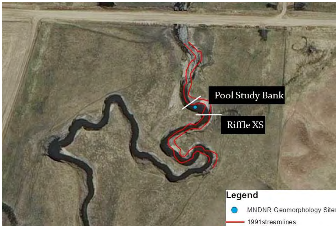
Figure 45. Aerial photo of the survey reach with labeled cross section locations and 1991 stream lines.
