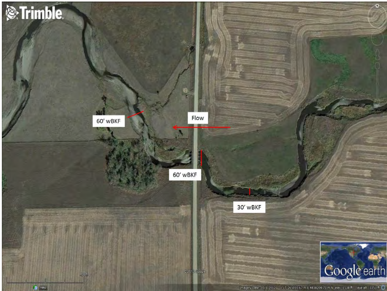
Figure 21. Aerial imagery of an oversized culvert on Kanaranzi Creek. The stream is flowing from right to left. Upstream of the culvert, the bankfull width is approximately 30 feet. The 4-barrel culvert is approximately 60 feet wide, affecting downstream bankfull widths to be twice as wide as upstream. Improper sizing of culverts can cause an excess amount of sediment downstream resulting in loss of habitat quality for a long distance downstream. Culverts should be properly sized to fit the bankfull channel and have flood relief culverts in the floodplain to handle high flows. Photo courtesy of Google Earth.
