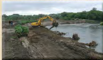
Installation of root wads using an excavator to drive tree trunks into the bankfull bench (looking upstream).
