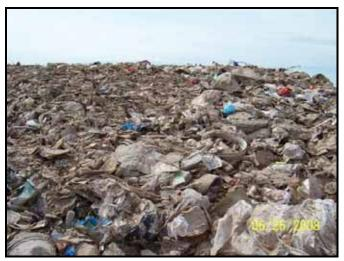
Example of inadequate application of cover material
