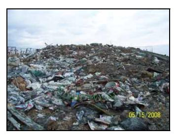
Example of inadequate application of cover material
