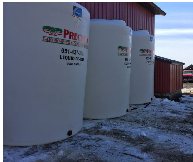
Liquid deicer storage tanks
