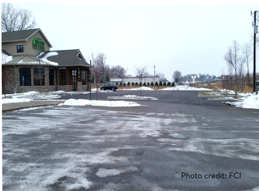
Figure 4-12 If your parking lot looks like this, too much salt was applied.
