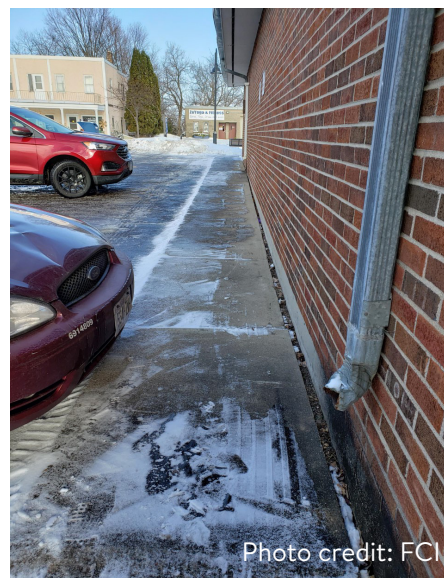
Figure 4-6 This downspout is an example of poor drainage causing ice.
