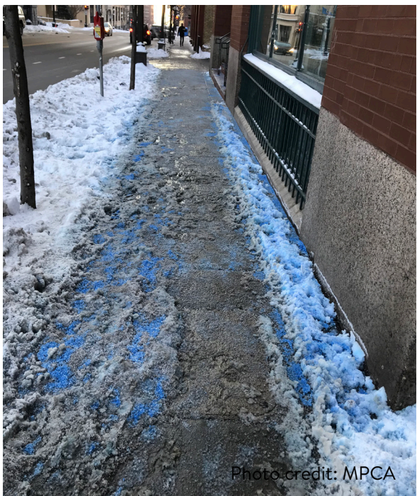
Figure 4-14 Too much salt and spread too far to the edges of the pavement.
