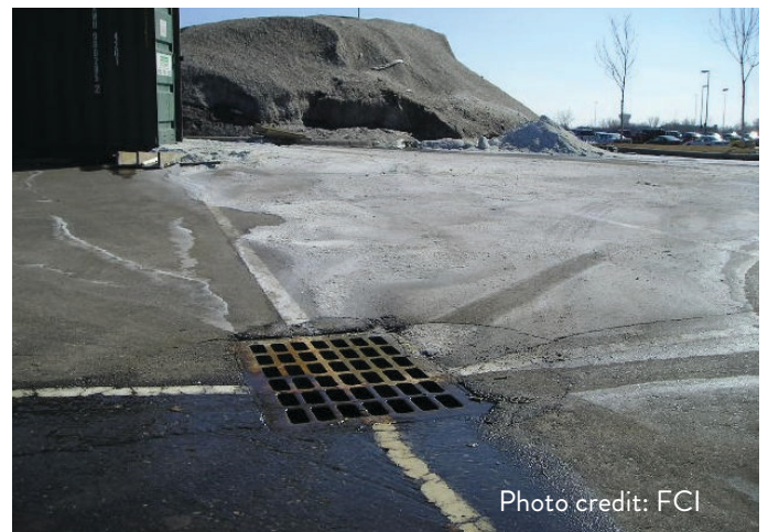
Figure 12: Incorrect salt storage: uncovered and placed in path of melting snow pile.
