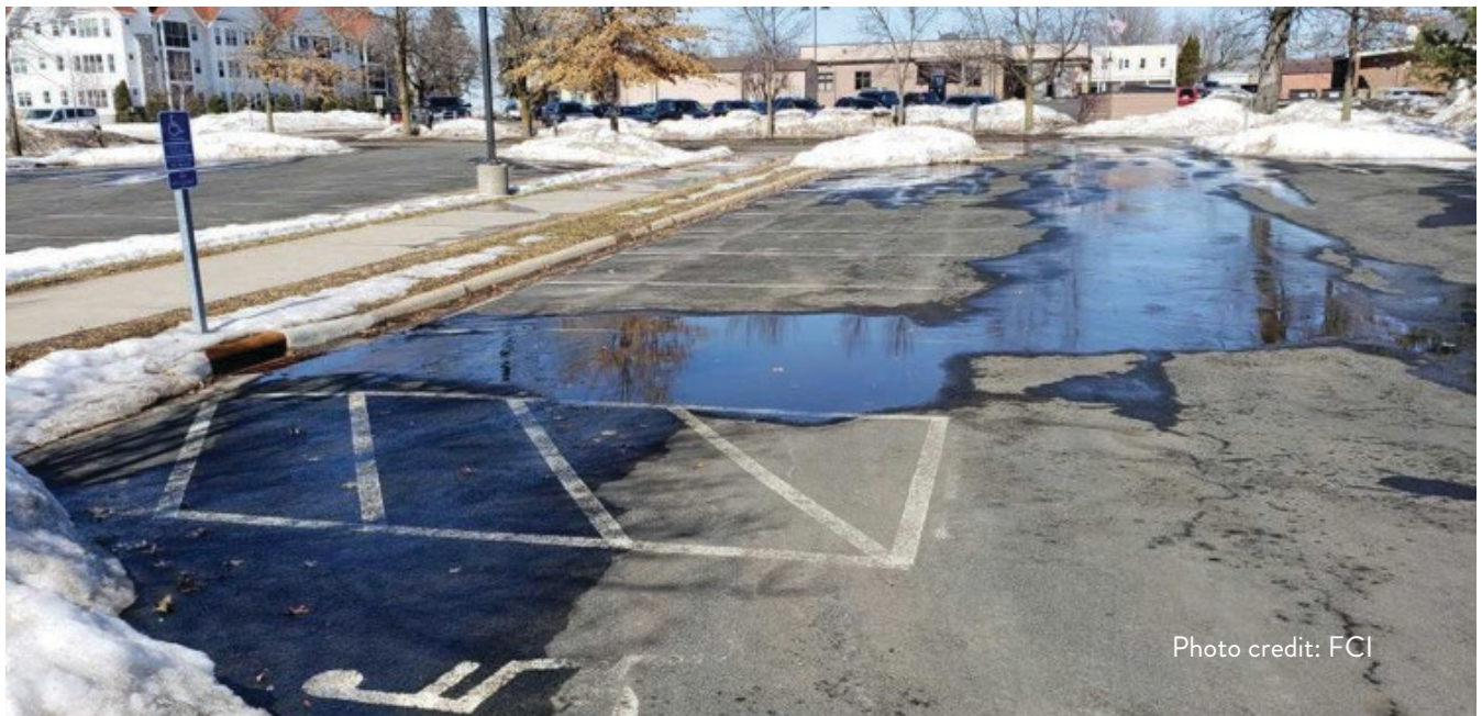
Figure 17: Poor design, handicap parking spot at storm drain.
