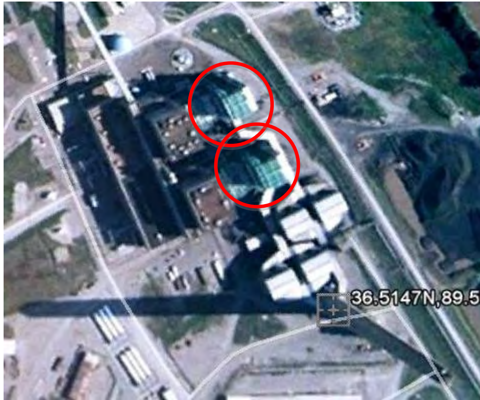
Figure 6-4. Site Layout for Associated Electric Cooperative's New Madrid Station, Units 1 and 2. (SCR reactors denoted within red circle)
