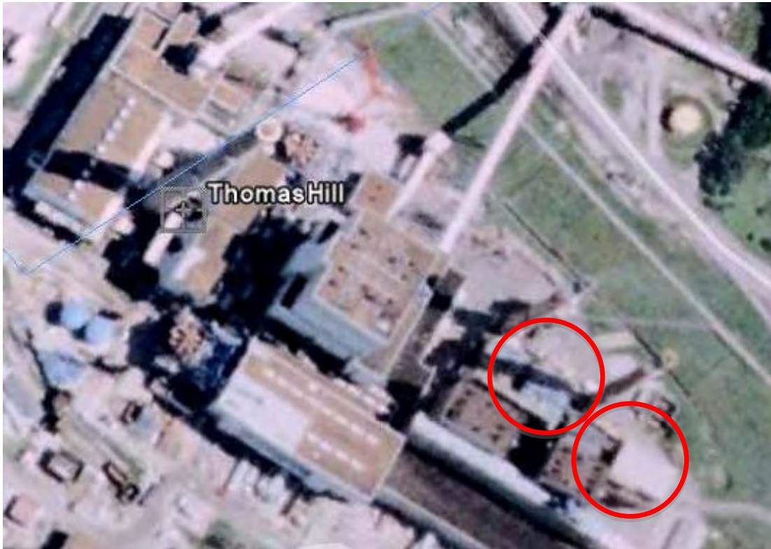
Figure 6-5. Site Layout for Associated Electric Cooperative’s Thomas Hill Station, Units 1 and 2. (SCR reactors denoted within red circle)
