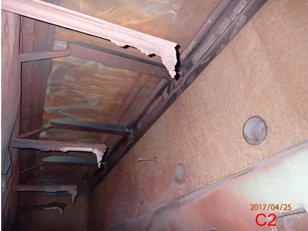
Photo 75 Scrubber C Mid-body (6)
