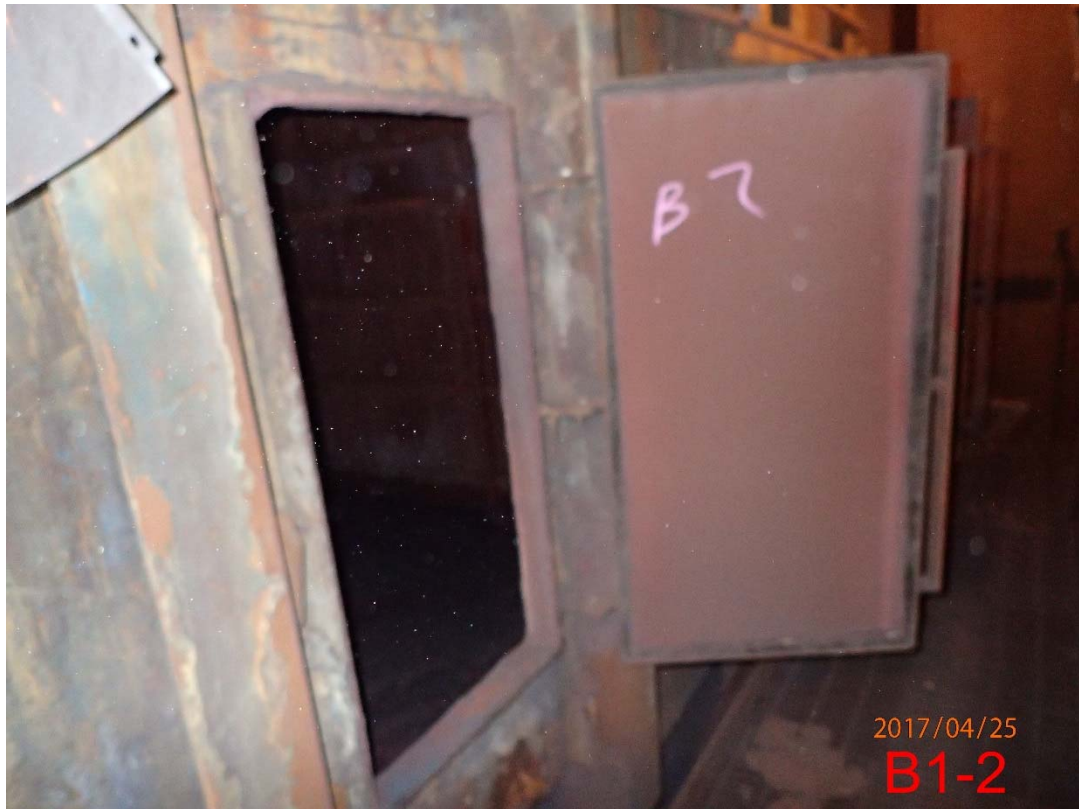
Photo 34 Transition Area from Scrubbers to Stack B (1)
