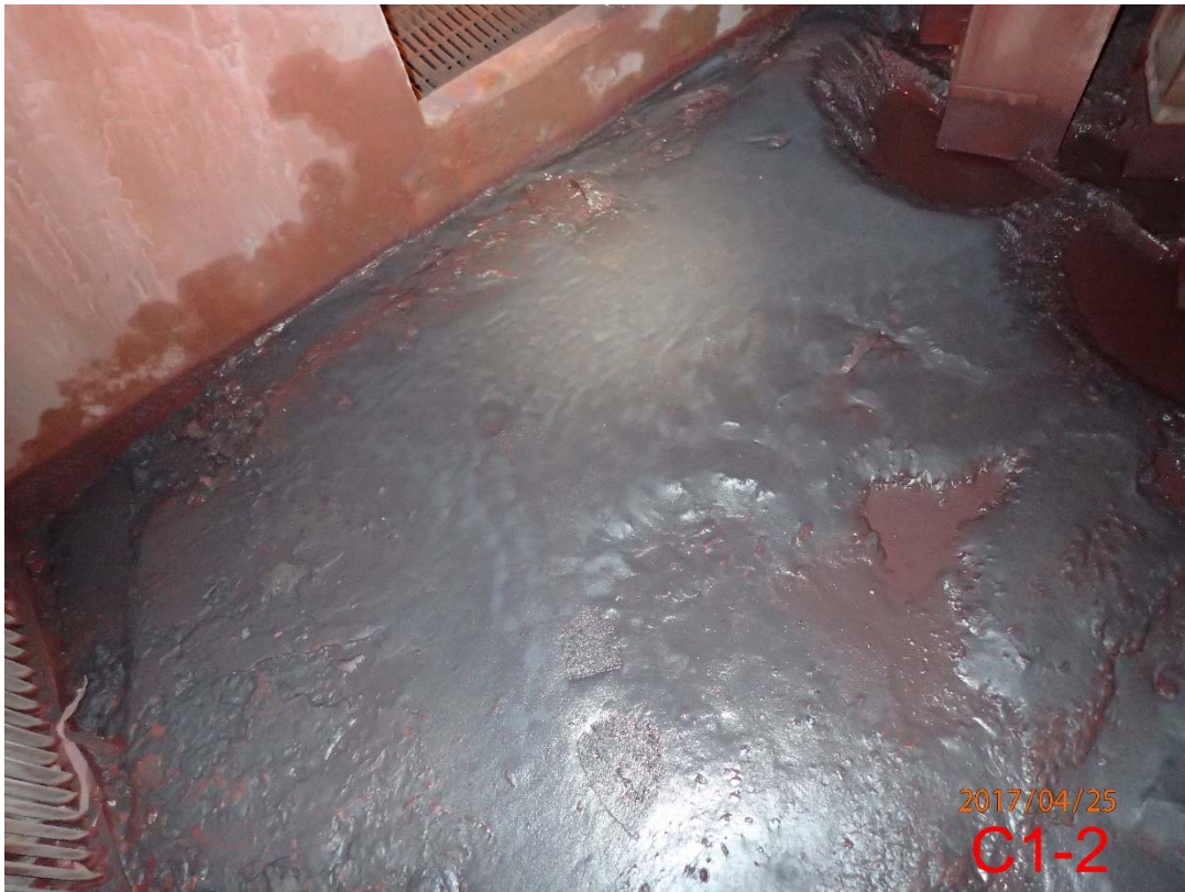
Photo 66 Transition Area from Scrubbers to Stack C (4)
