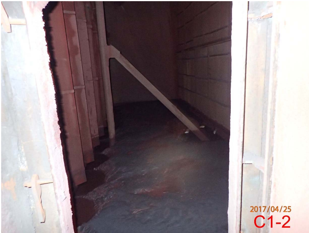
Photo 64 Transition Area from Scrubbers to Stack C (2)
