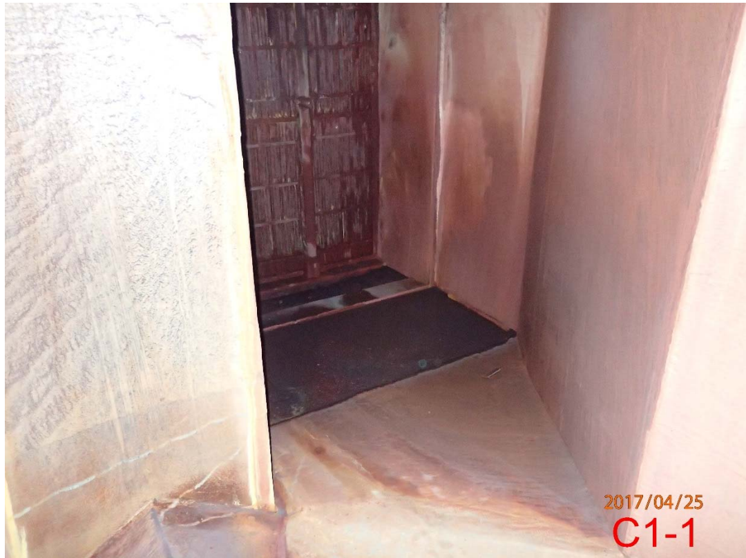
Photo 60 Base of Stack C (10)
