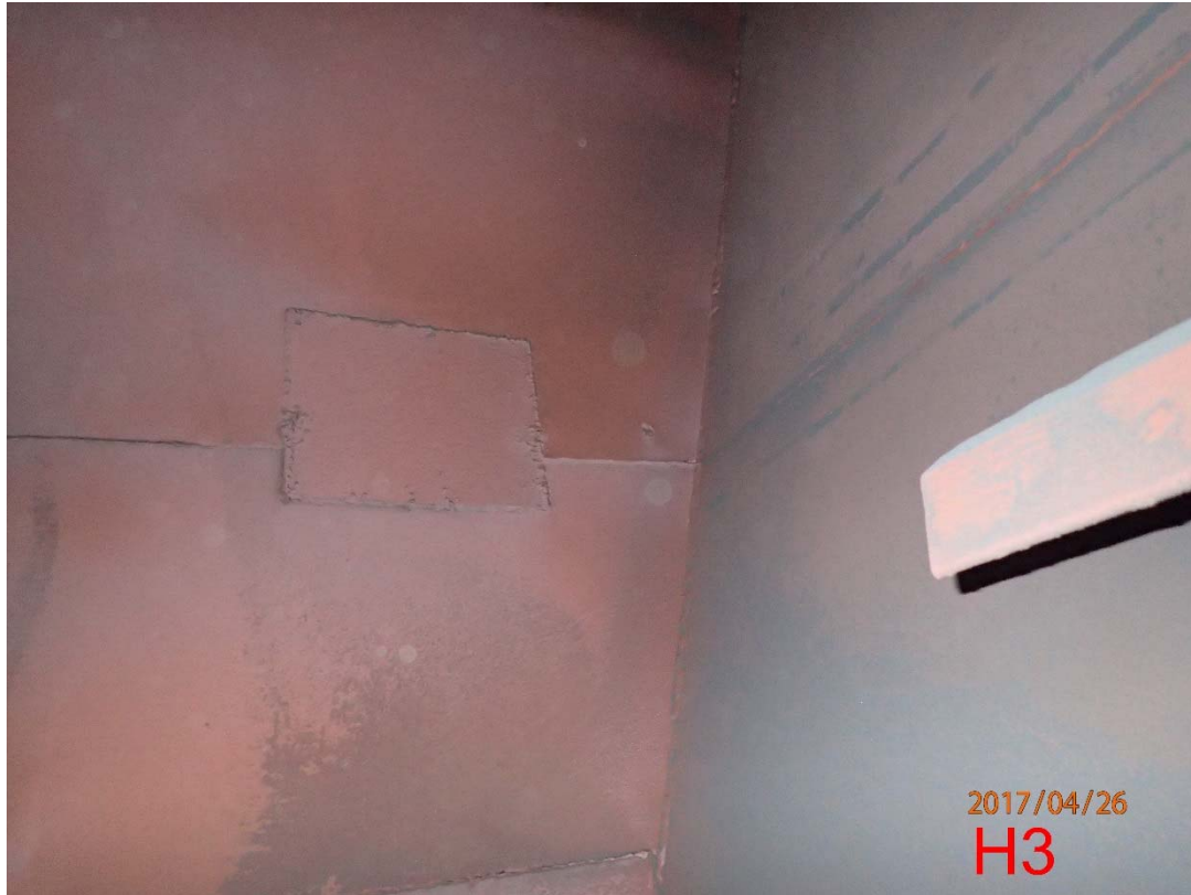
Photo 145 Multiclone Cones at Second Level (18)
