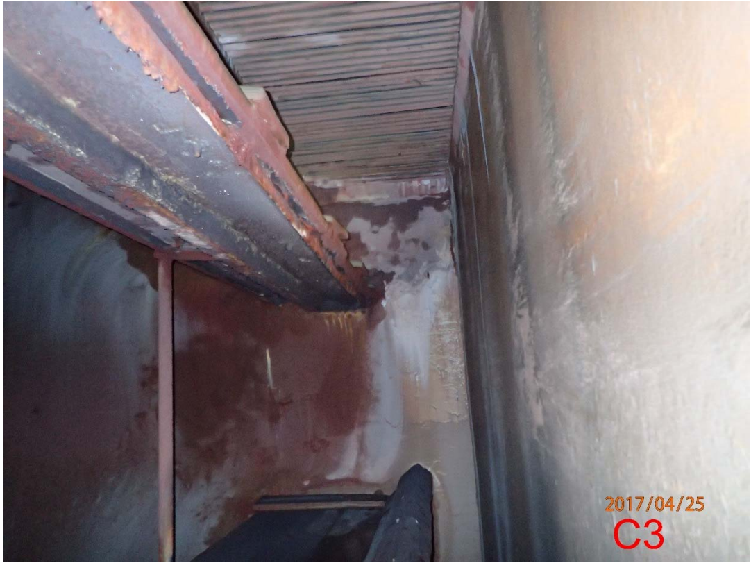
Photo 80 Scrubber C Lower-body (5)
