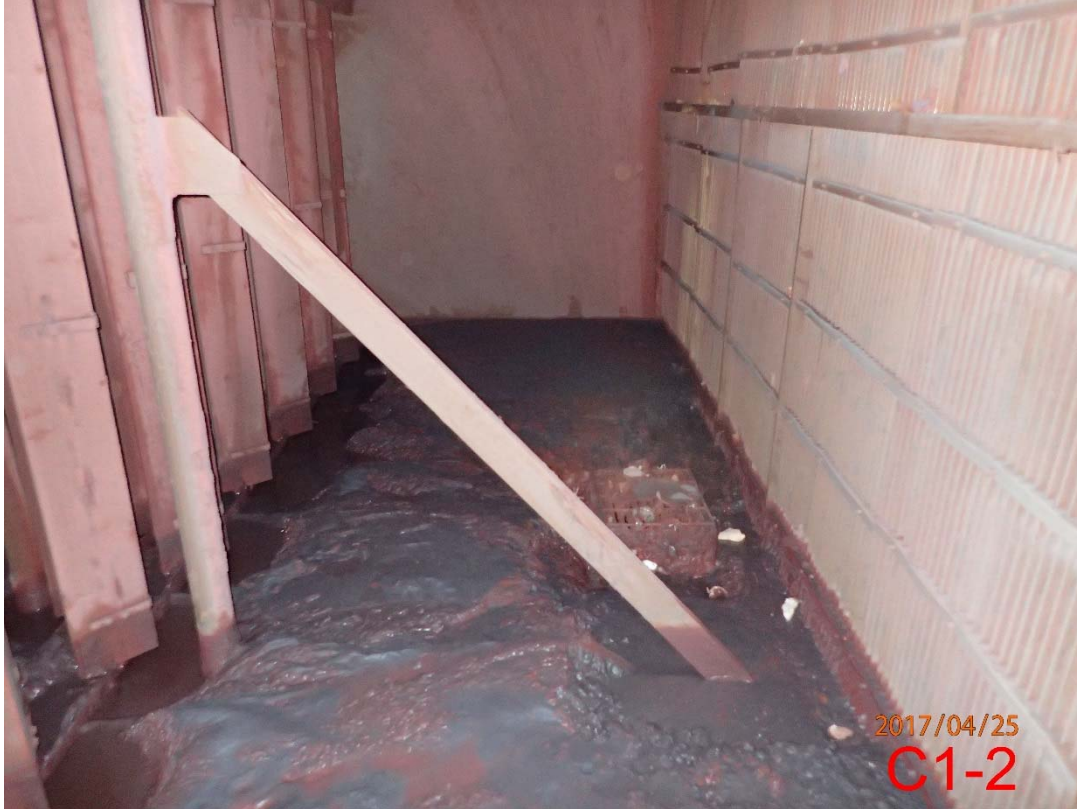
Photo 67 Transition Area from Scrubbers to Stack C (5)
