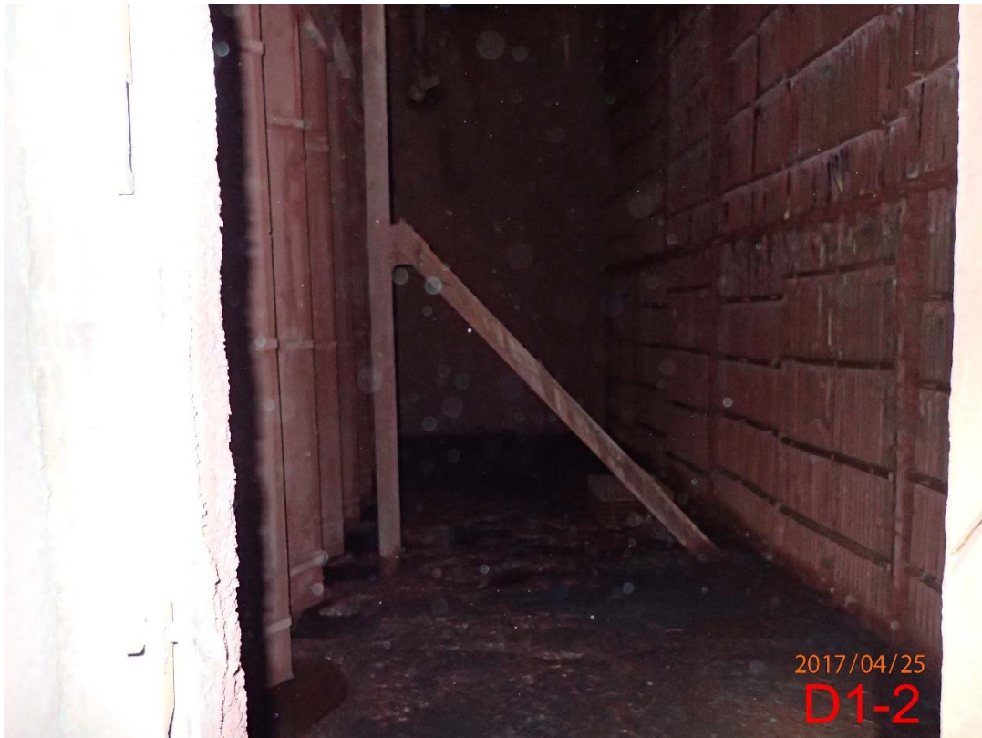
Photo 90 Transition Area from Scrubbers to Stack D (2)
