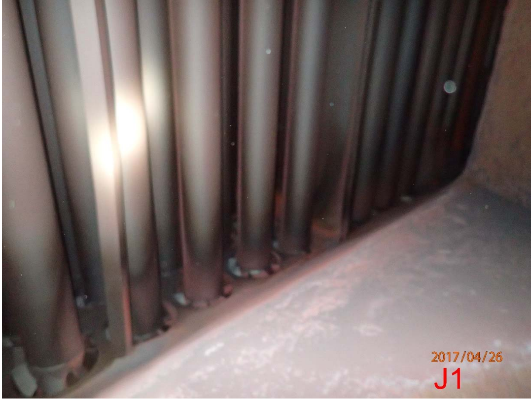
Photo 157 Ducting off Process Gas Header (4)
