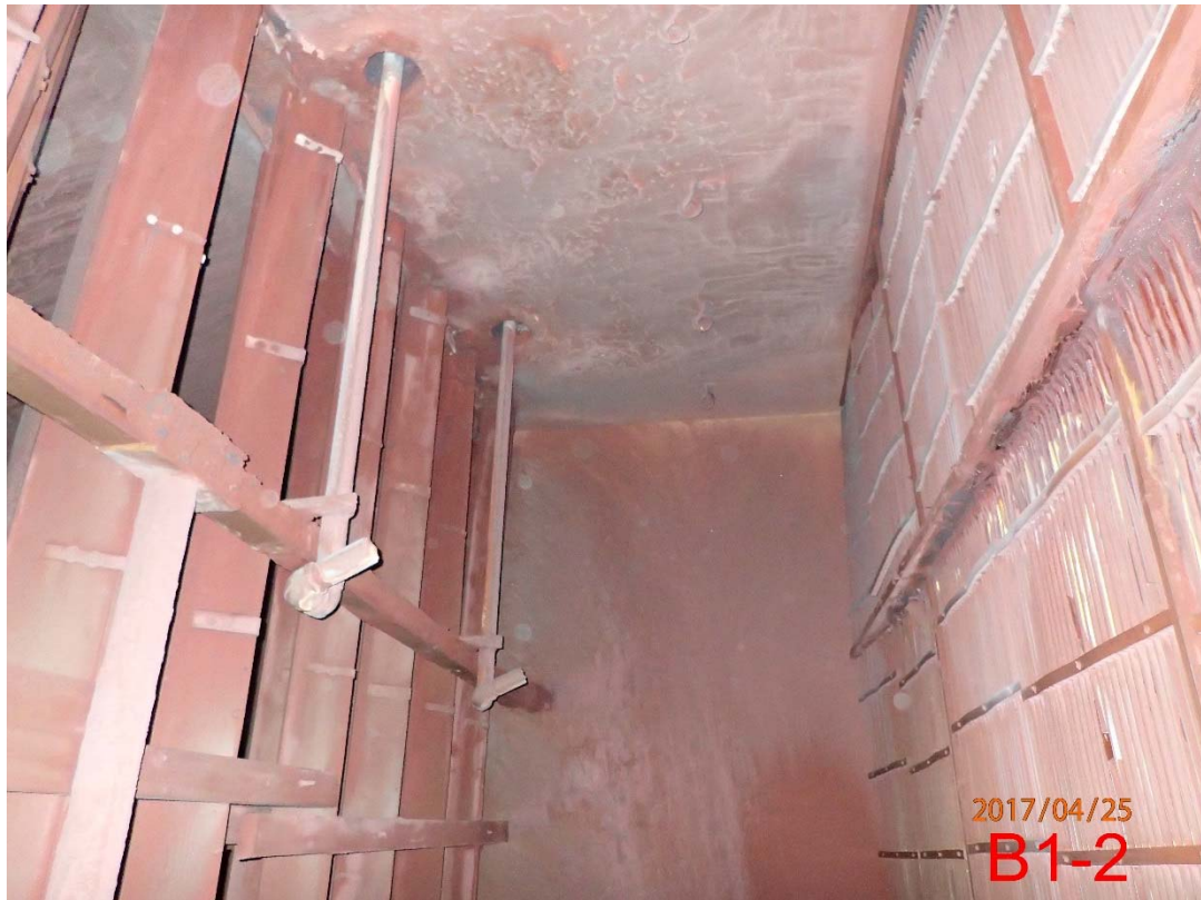
Photo 36 Transition Area from Scrubbers to Stack B (3)
