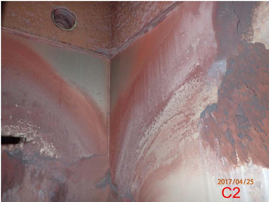
Photo 72 Scrubber C Mid-body (3)
