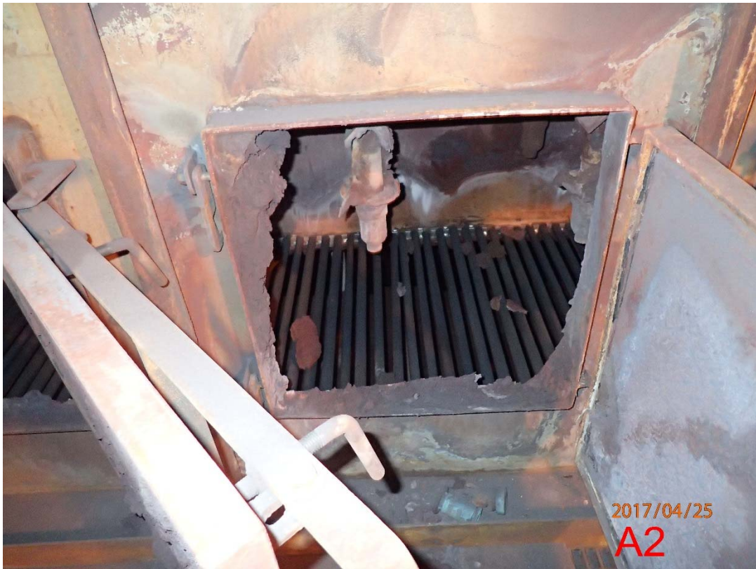
Photo 14 Scrubber A Mid-body (3)
