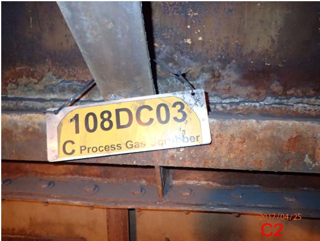
Photo 70 Scrubber C Mid-body (1)
