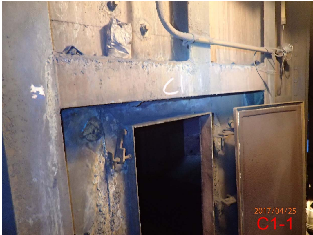
Photo 51 Base of Stack C (1)
