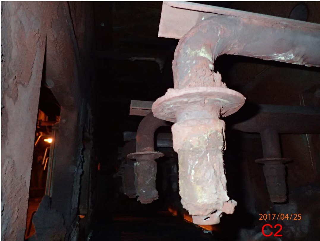
Photo 74 Scrubber C Mid-body (5)
