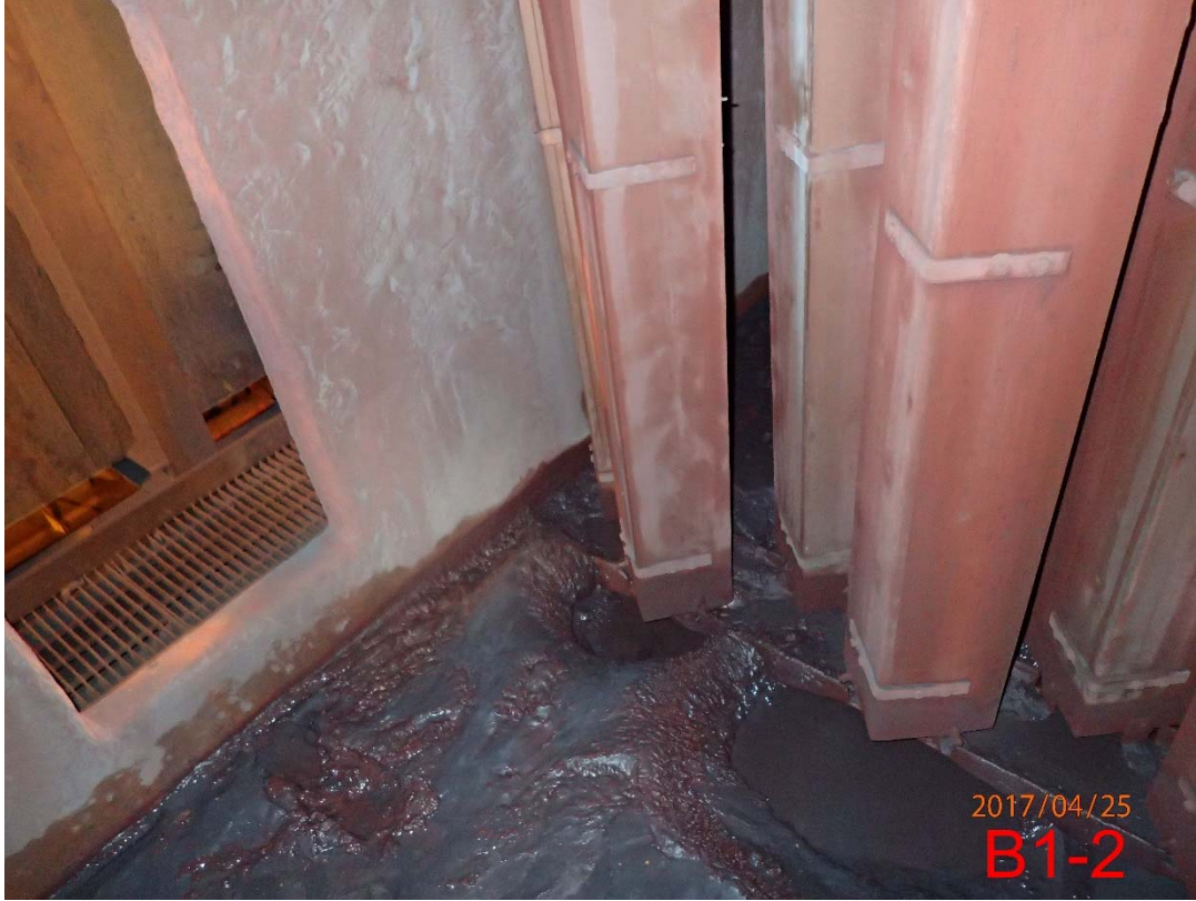
Photo 39 Transition Area from Scrubbers to Stack B (6)
