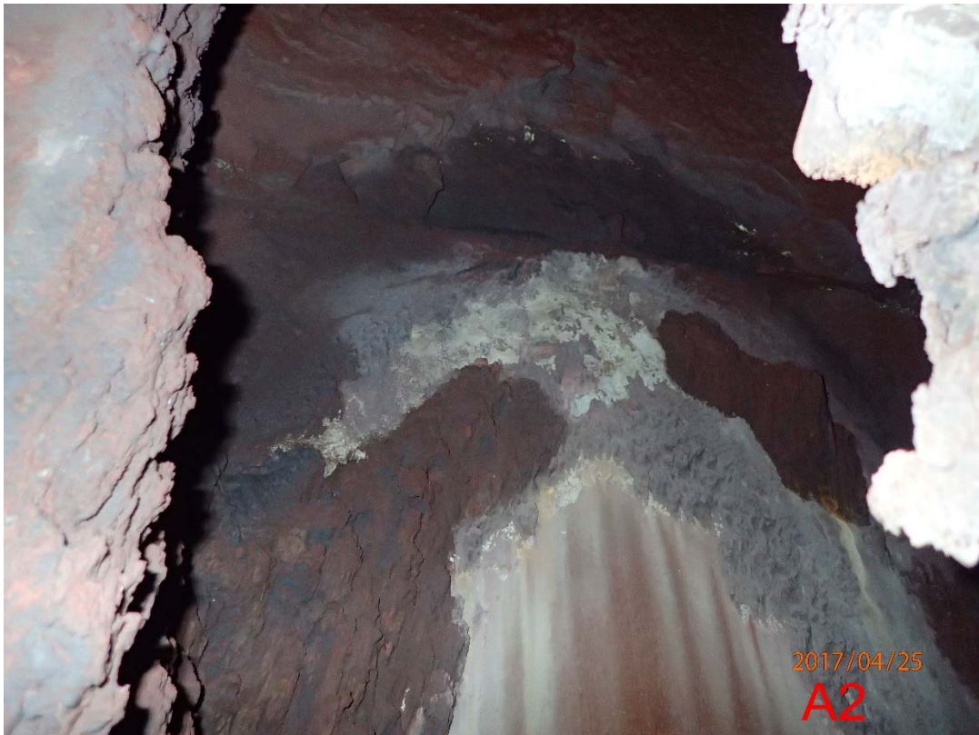
Photo 16 Scrubber A Mid-body (5)
