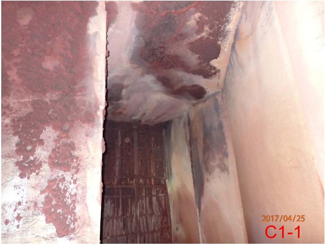
Photo 56 Base of Stack C (6)
