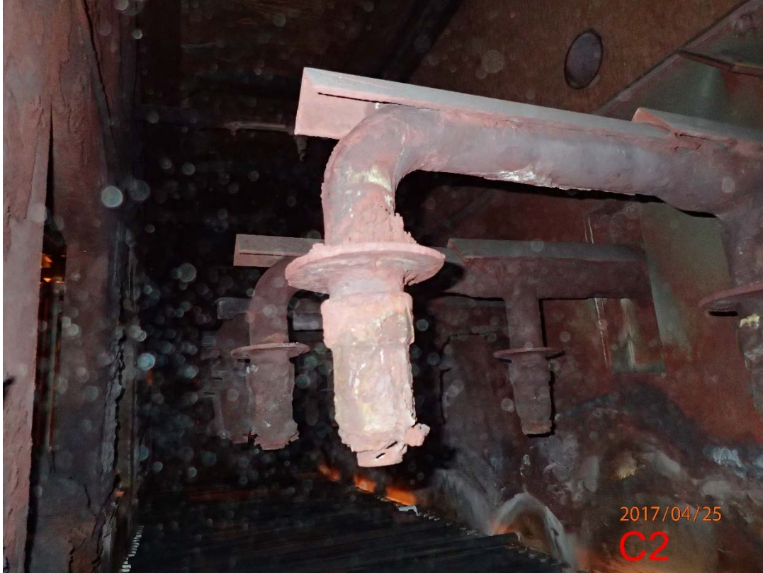
Photo 71 Scrubber C Mid-body (2)
