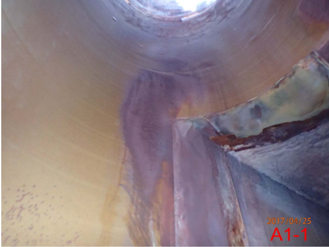
Photo 7 Base of Stack A (7)
