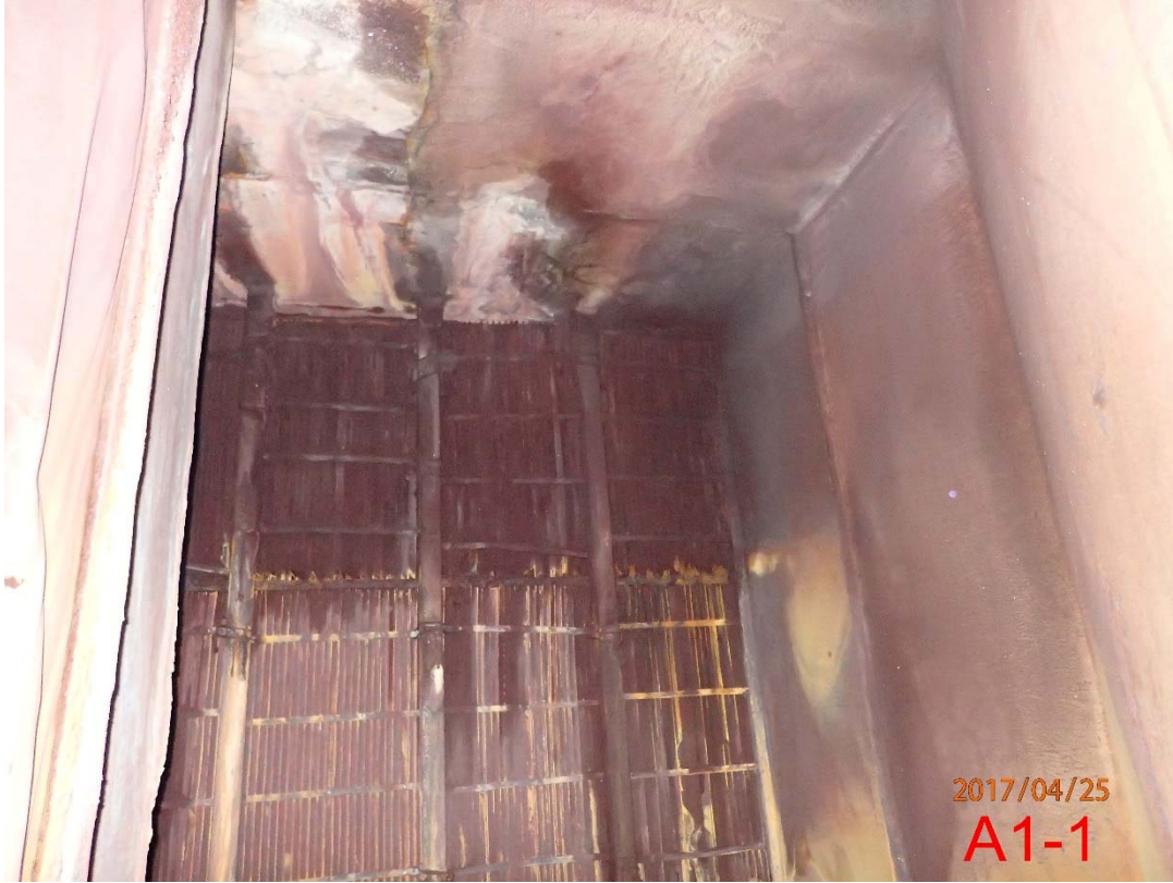
Photo 5 Base of Stack A (5)
