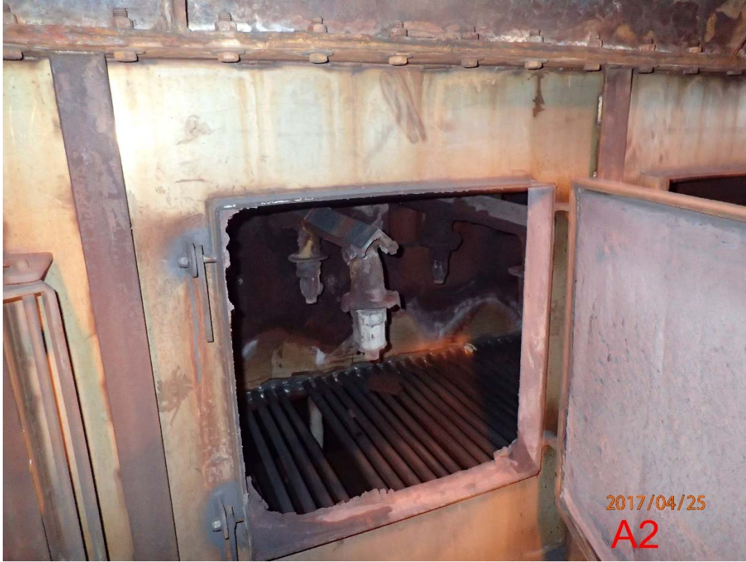
Photo 17 Scrubber A Mid-body (6)
