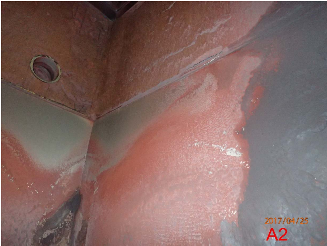
Photo 18 Scrubber A Mid-body (7)
