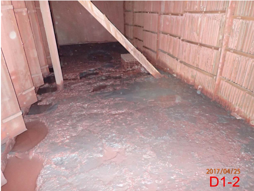
Photo 89 Transition Area from Scrubbers to Stack D (1)
