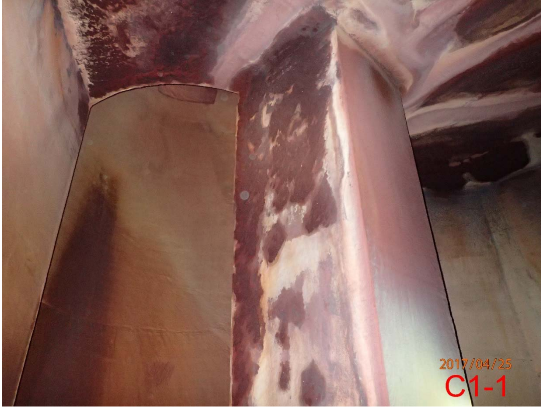
Photo 61 Base of Stack C (11)
