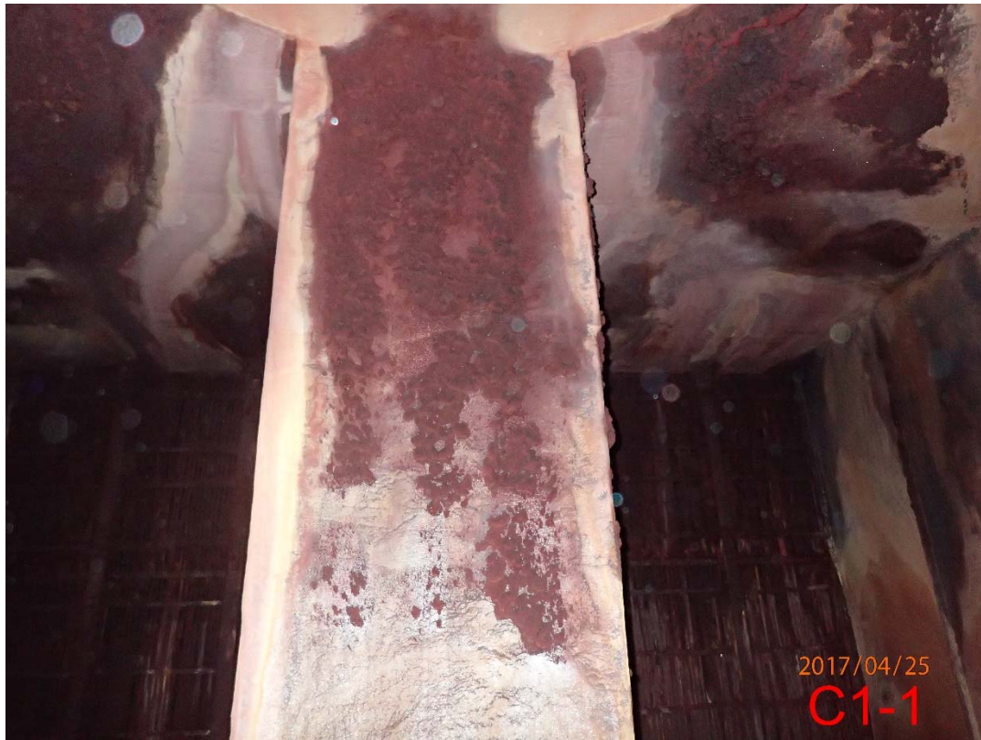
Photo 54 Base of Stack C (4)
