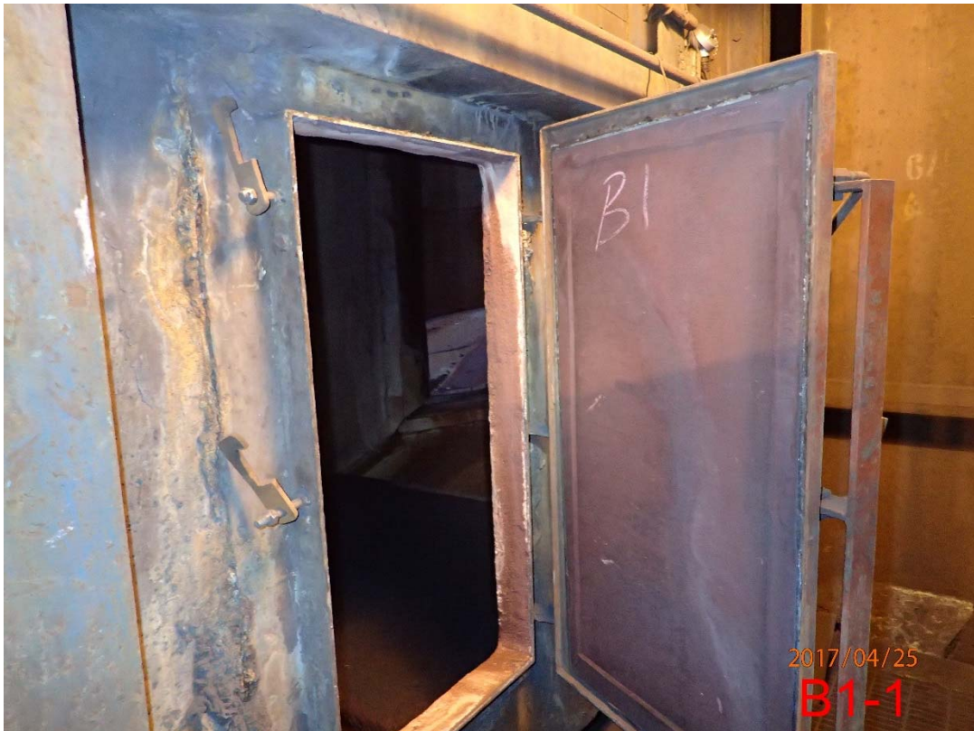
Photo 26 Base of Stack B (1)
