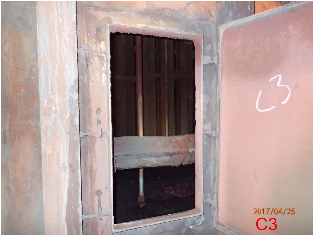
Photo 76 Scrubber C Lower-body (1)
