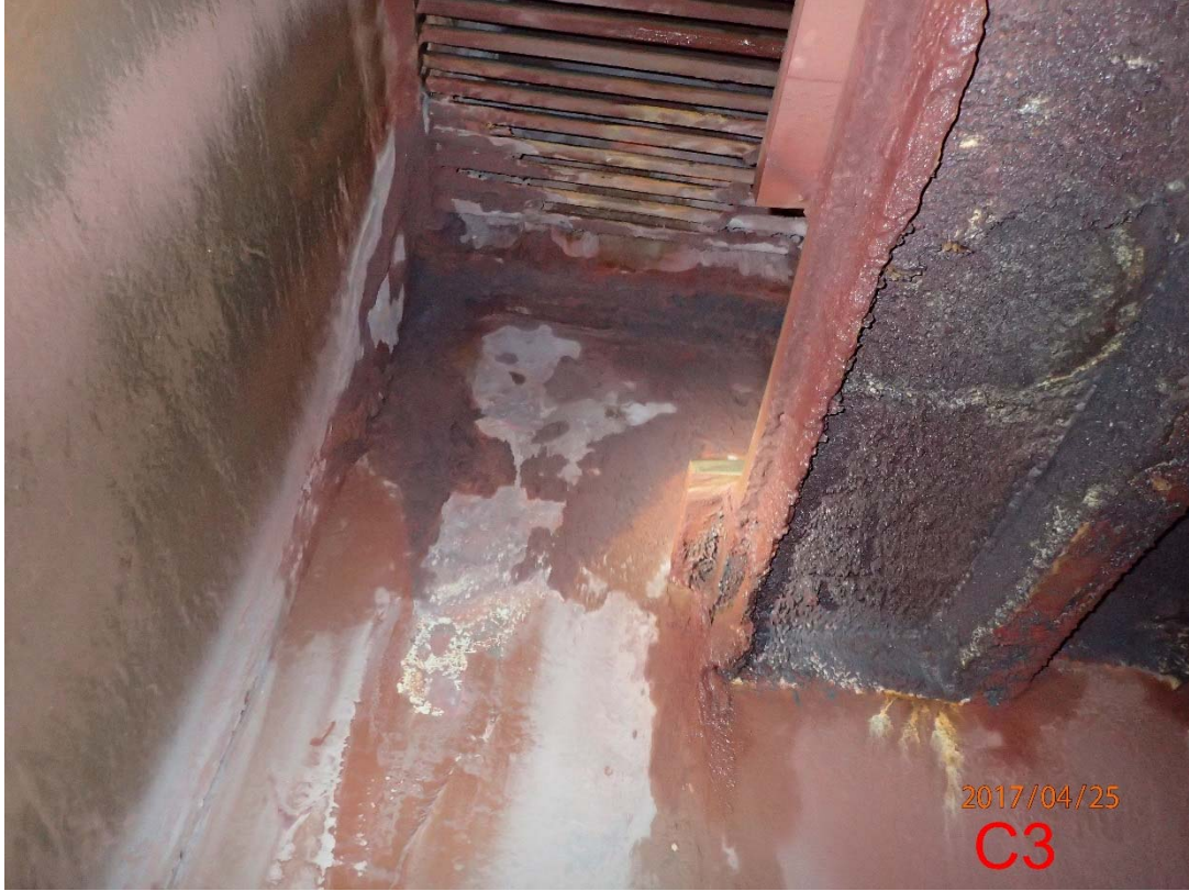
Photo 79 Scrubber C Lower-body (4)
