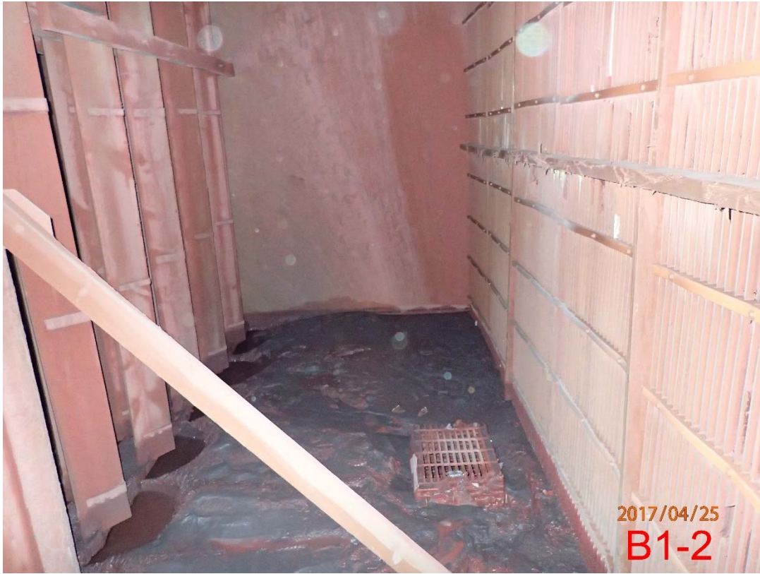
Photo 37 Transition Area from Scrubbers to Stack B (4)
