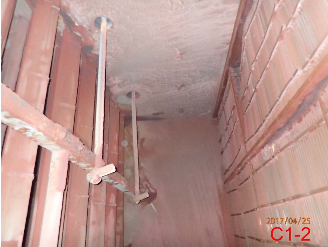
Photo 65 Transition Area from Scrubbers to Stack C (3)
