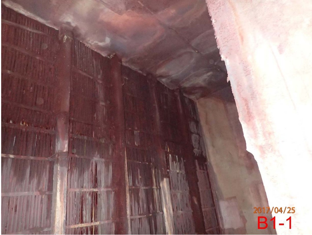
Photo 27 Base of Stack B (2)
