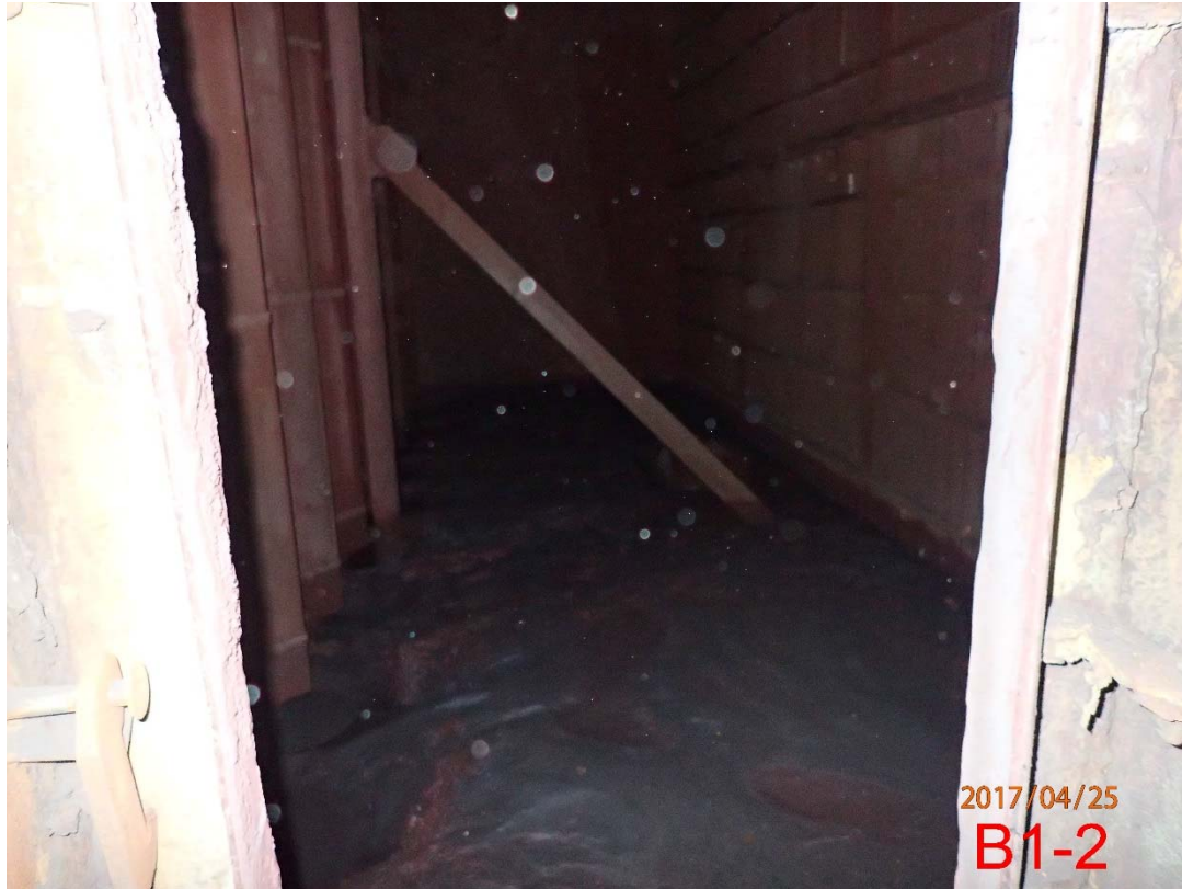
Photo 35 Transition Area from Scrubbers to Stack B (2)
