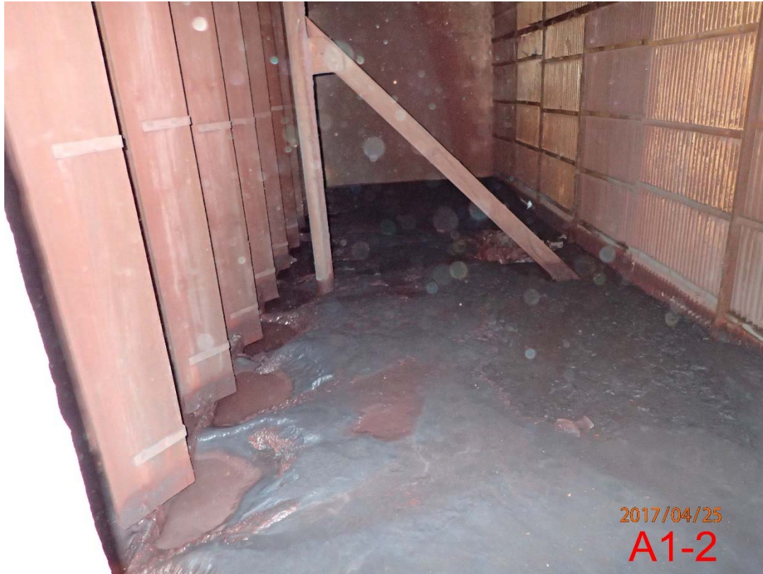
Photo 9 Transition Area from Scrubbers to Stack A (2)
