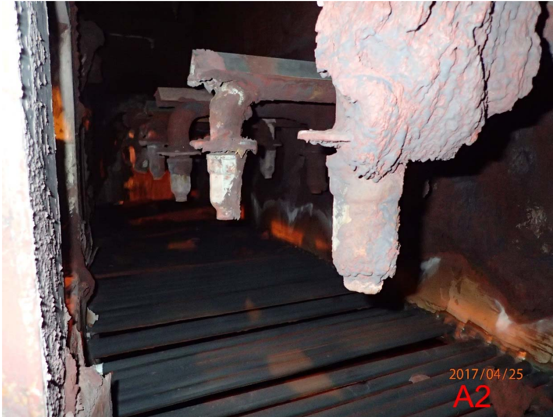
Photo 19 Scrubber A Mid-body (8)
