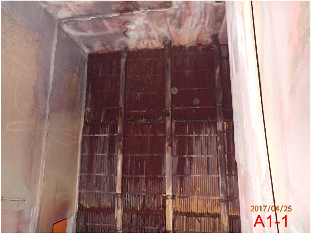
Photo 4 Base of Stack A (4)
