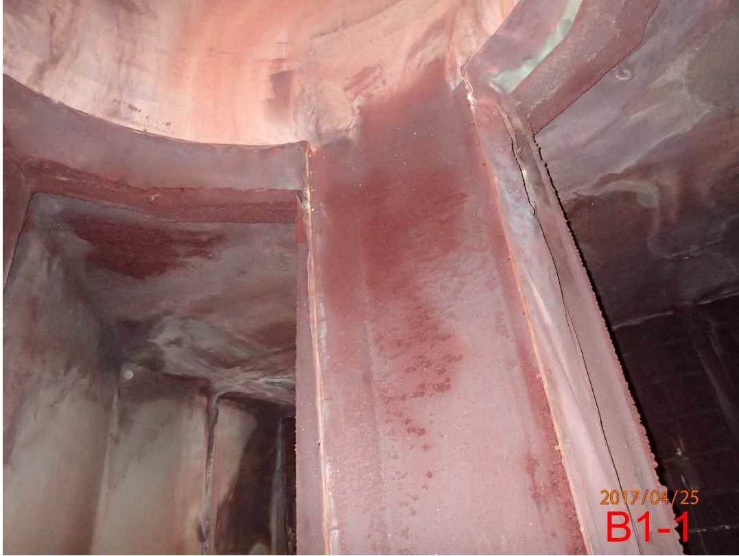
Photo 31 Base of Stack B (6)
