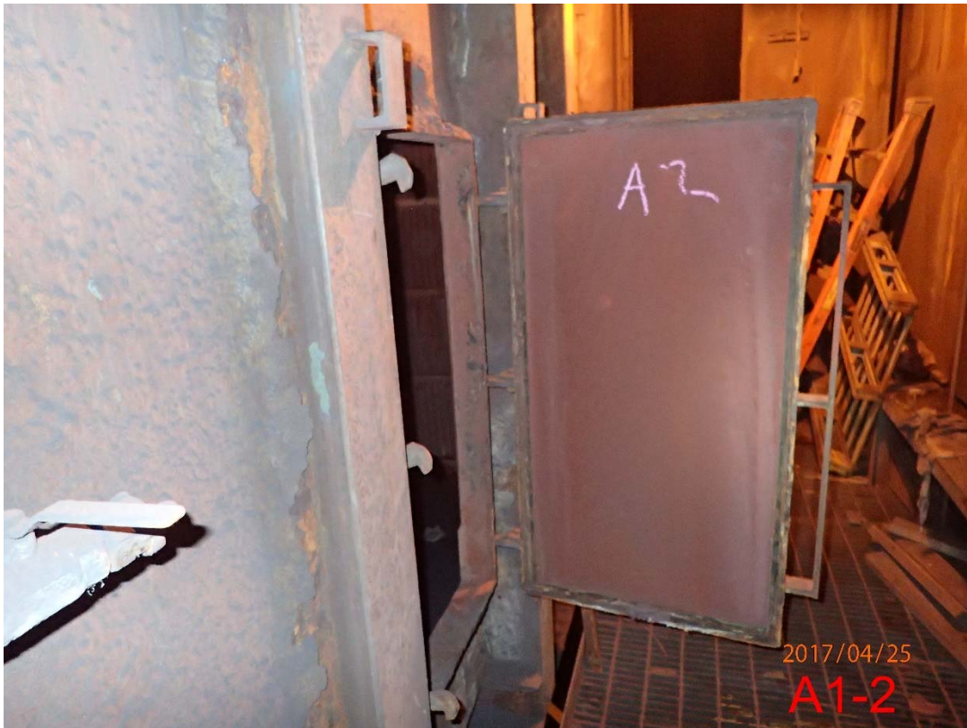
Photo 8 Transition Area from Scrubbers to Stack A (1)
