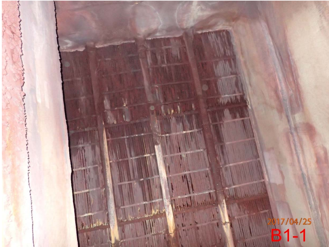
Photo 33 Base of Stack B (8)
