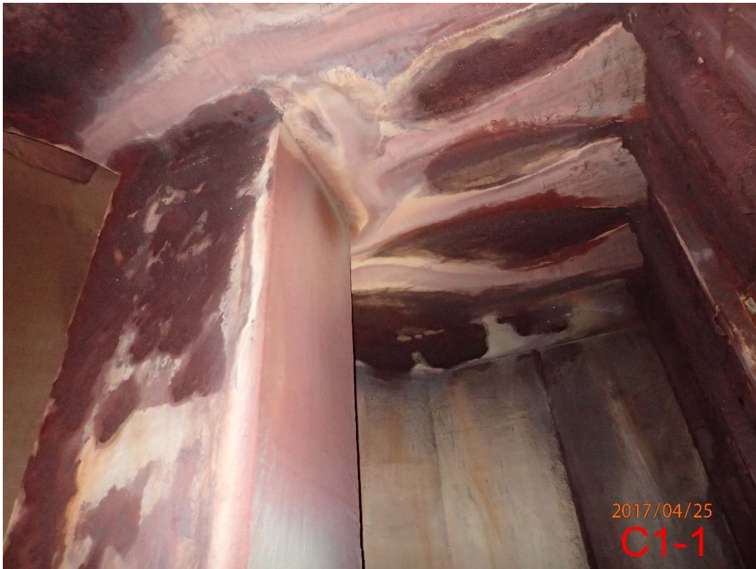
Photo 62 Base of Stack C (12)
