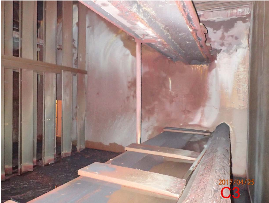
Photo 77 Scrubber C Lower-body (2)
