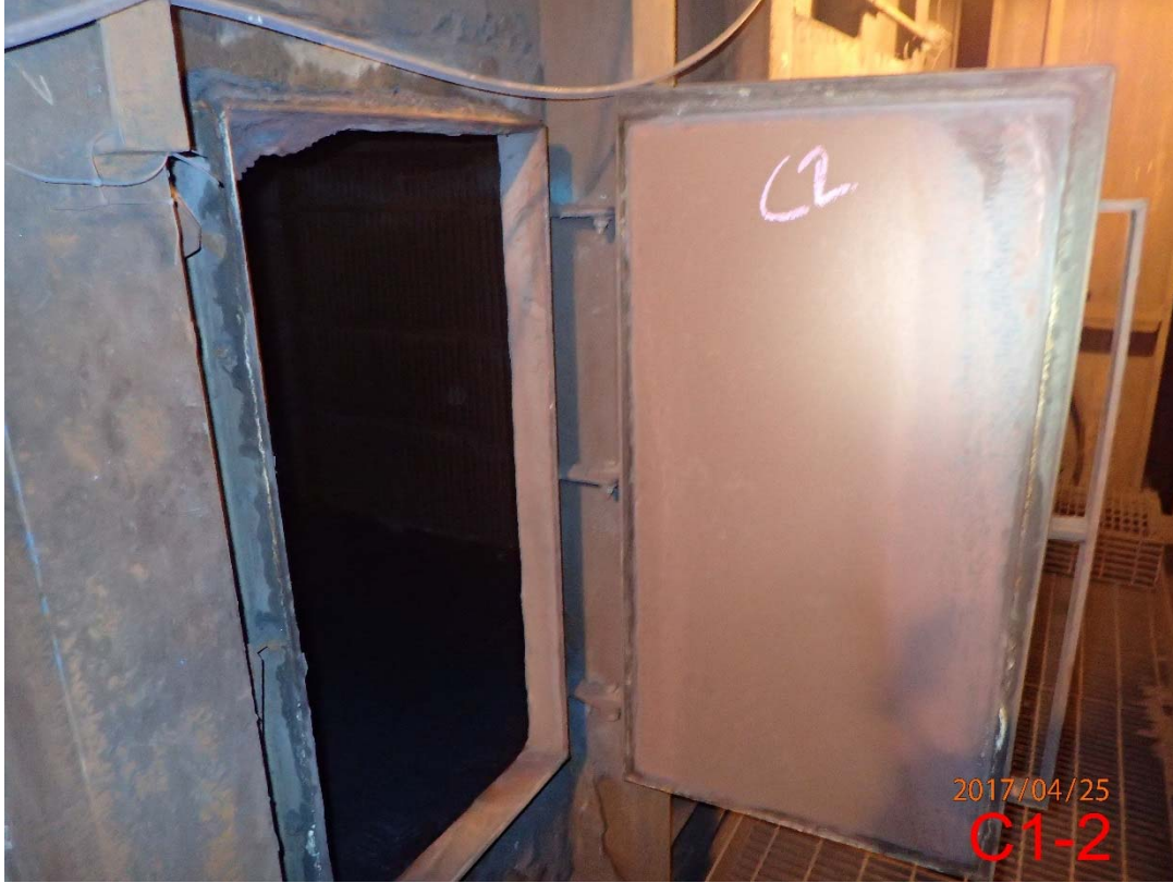
Photo 63 Transition Area from Scrubbers to Stack C (1)
