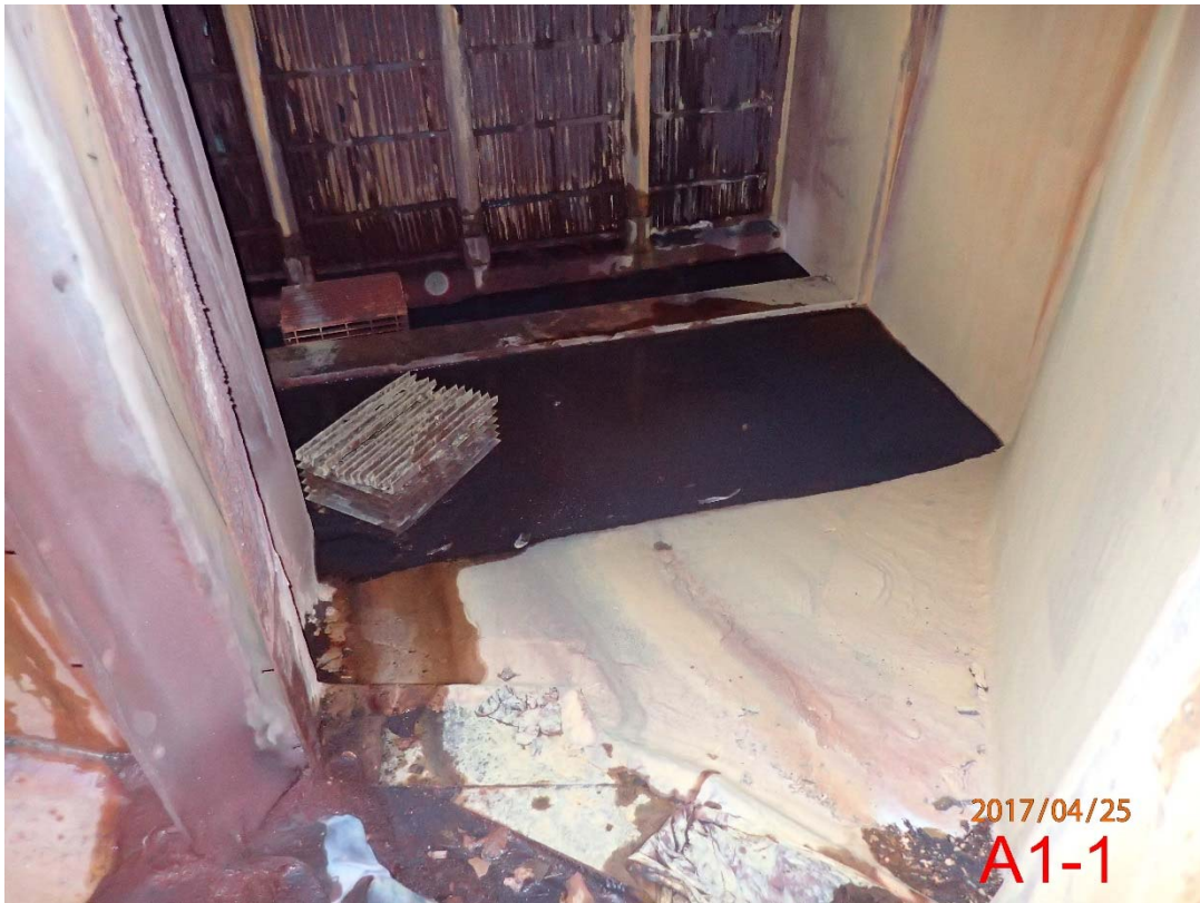
Photo 6 Base of Stack A (6)
