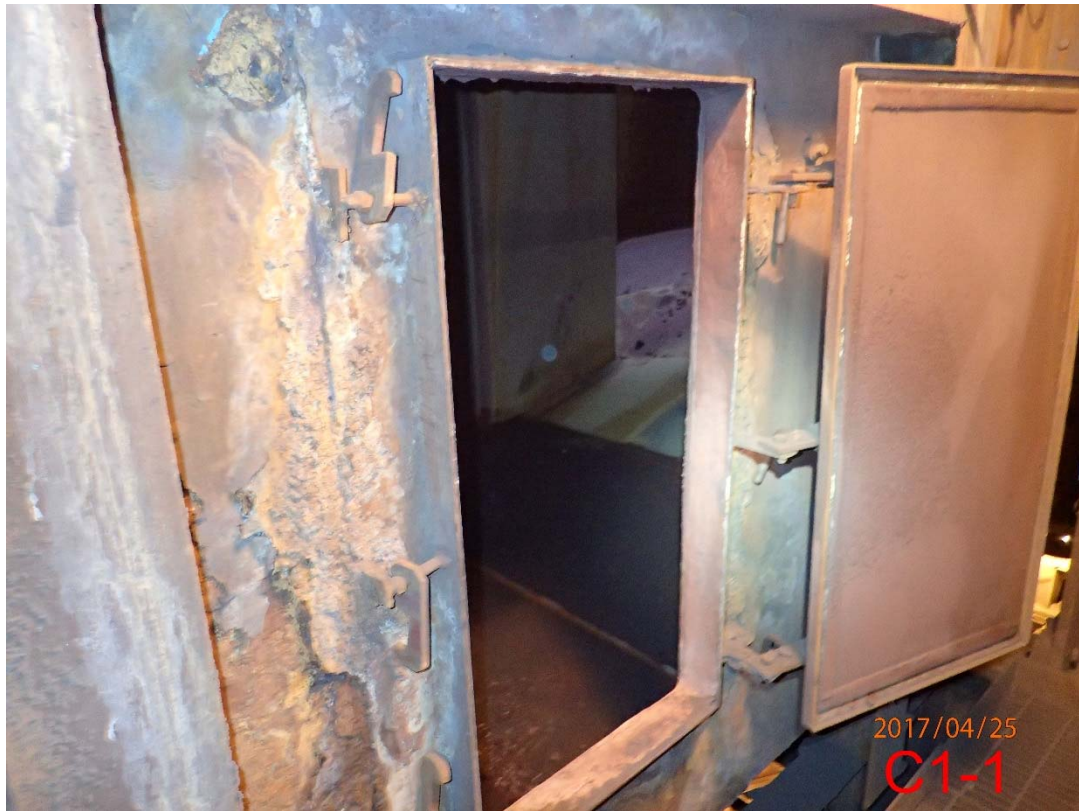
Photo 52 Base of Stack C (2)
