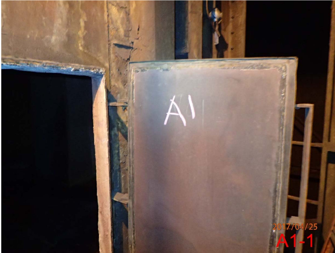
Photo 1 Base of Stack A (1)
