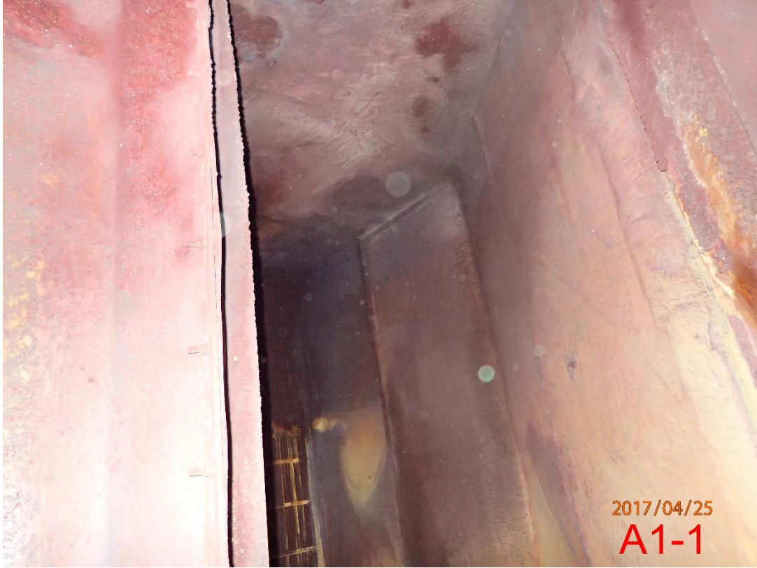
Photo 3 Base of Stack A (3)
