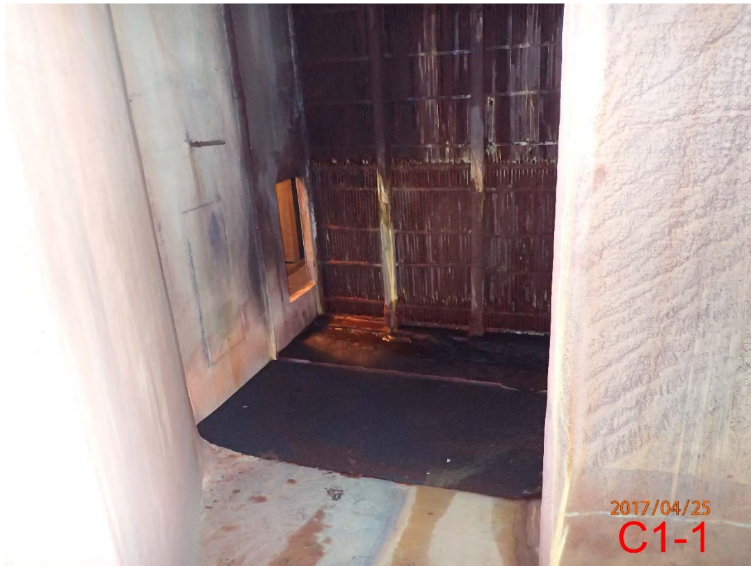
Photo 59 Base of Stack C (9)
