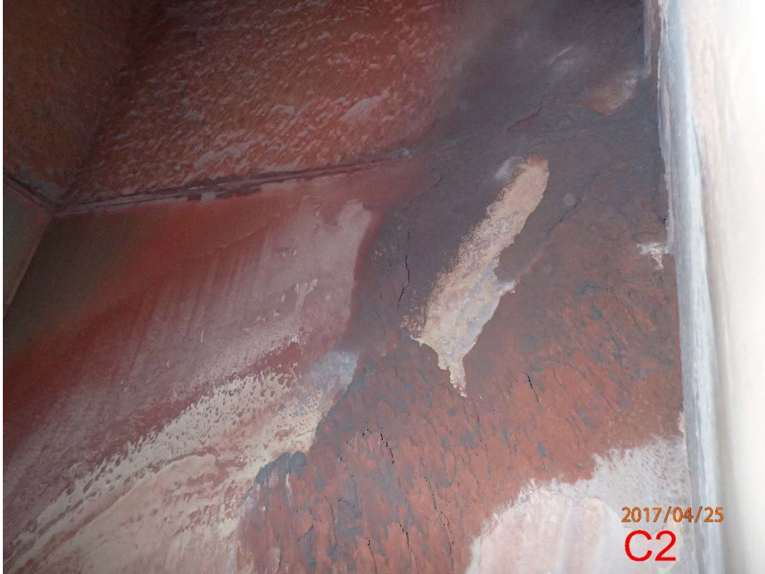
Photo 73 Scrubber C Mid-body (4)
