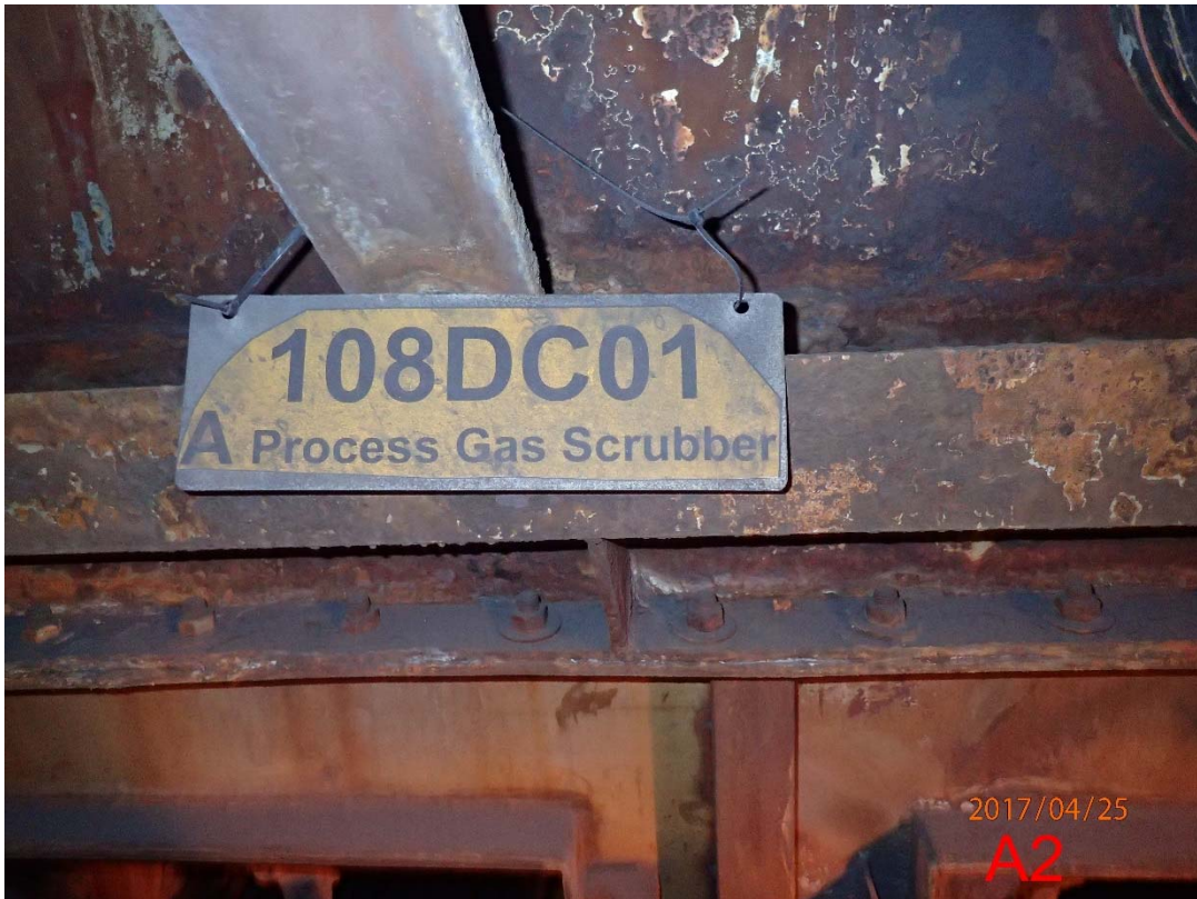
Photo 12 Scrubber A Mid-body (1)
