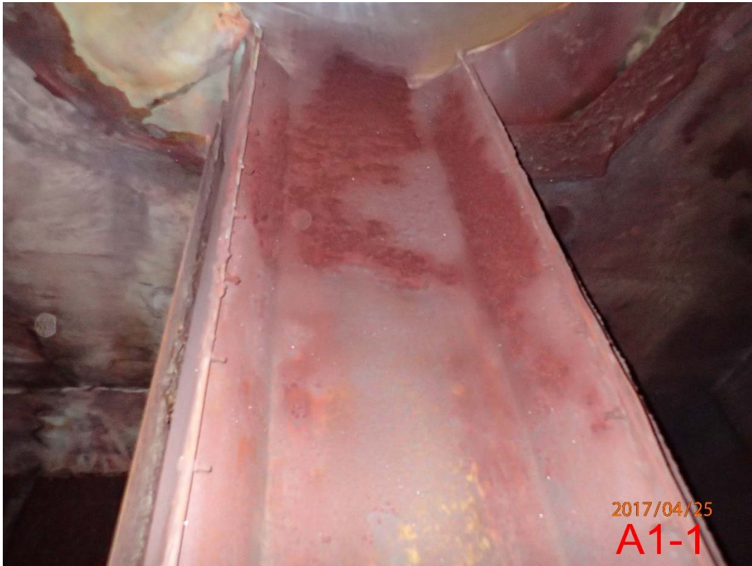
Photo 2 Base of Stack A (2)
