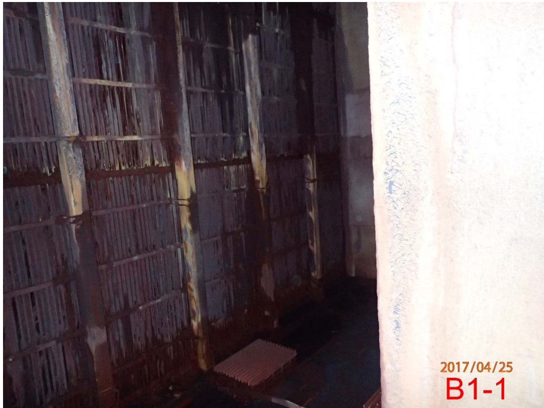
Photo 30 Base of Stack B (5)
