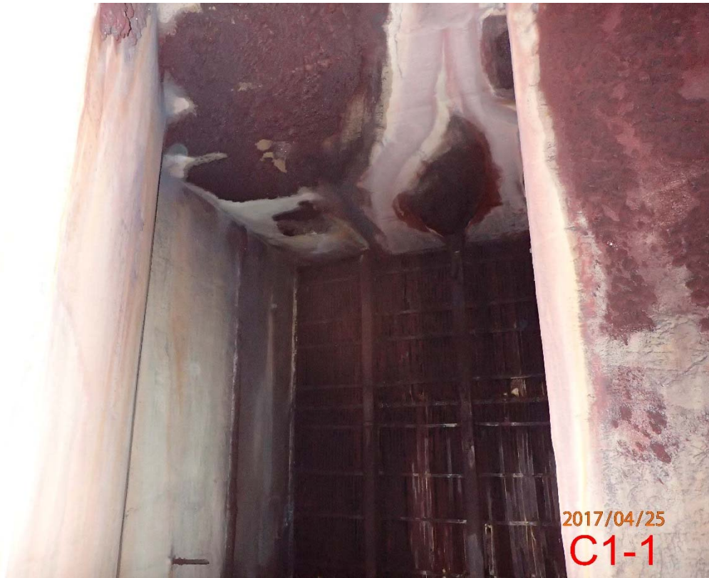
Photo 58 Base of Stack C (8)
