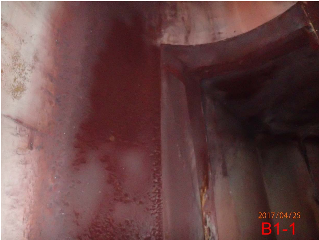
Photo 32 Base of Stack B (7)
