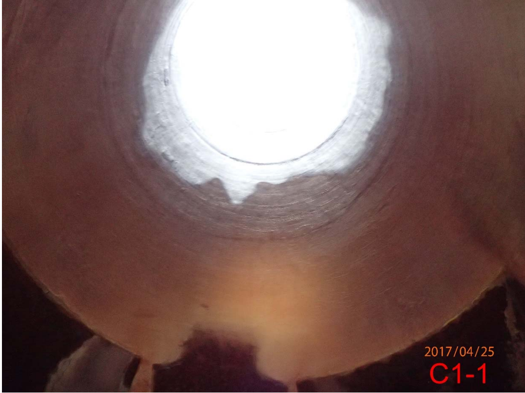
Photo 55 Base of Stack C (5)
