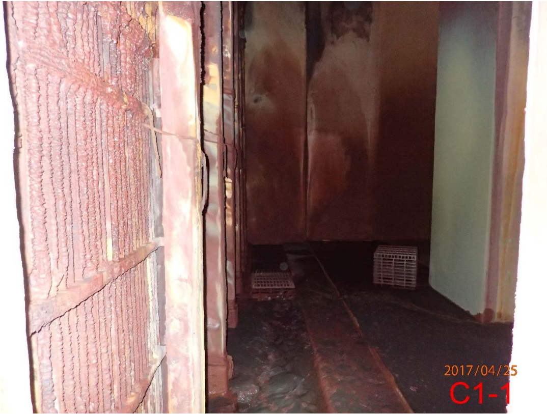
Photo 53 Base of Stack C (3)
