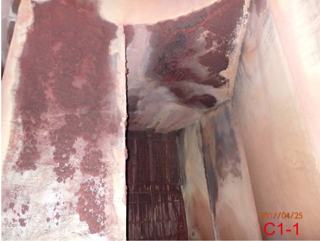
Photo 57 Base of Stack C (7)
