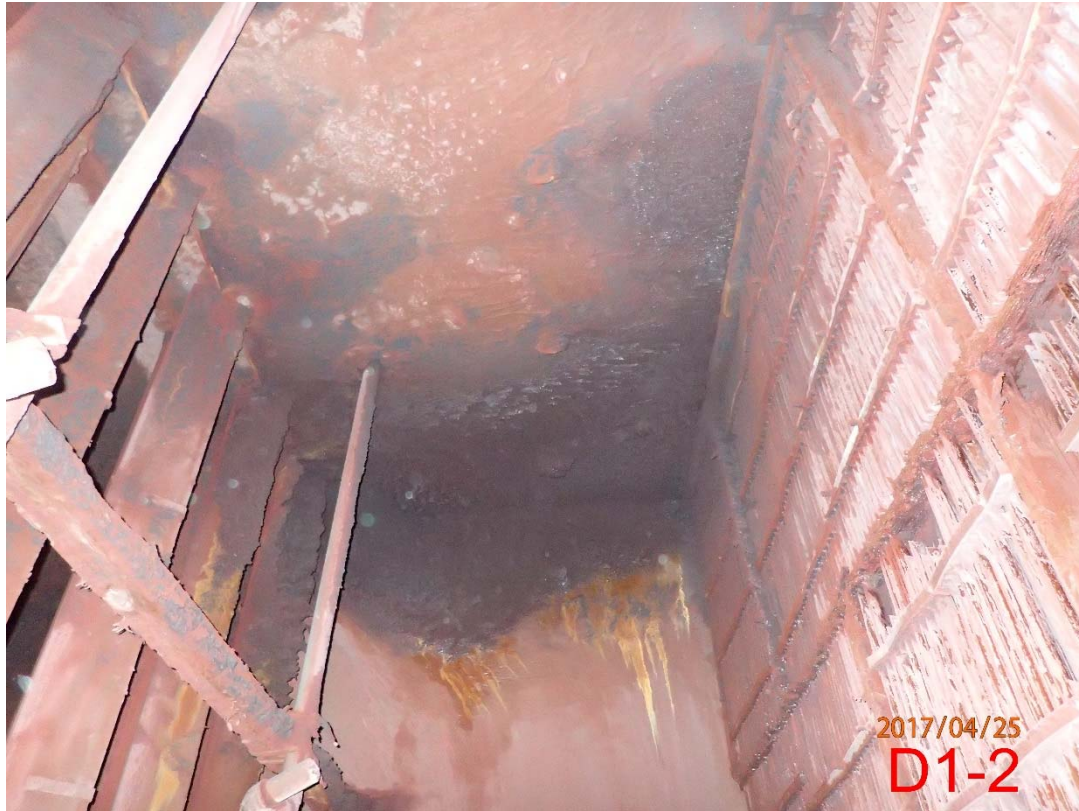
Photo 91 Transition Area from Scrubbers to Stack D (3)
