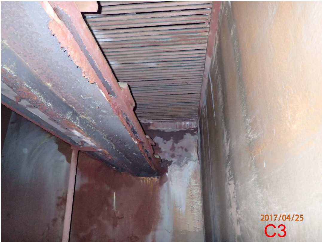
Photo 78 Scrubber C Lower-body (3)
