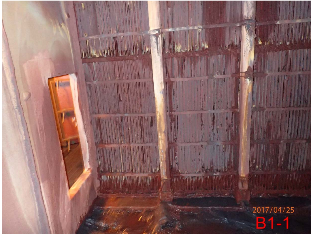
Photo 29 Base of Stack B (4)
