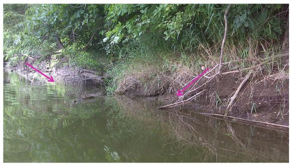
Figure 40. Fence posts that have fallen into the river from losing surrounding soil (8-4-11).
