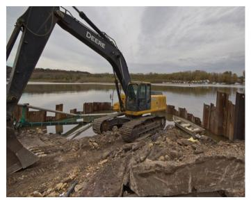
Coffer dams made of sheet metal to isolate the work area from the surface water.
