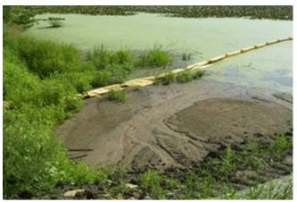
Relying on floating curtain as downgradient perimeter control will result in permit violations for failure to install sediment control and in most cases will result in water quality violations.
