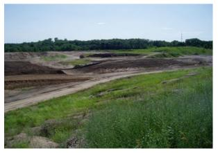
Slope tracking roughens the surface of a slope and decreases the velocity of runoff.
