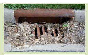
A storm drain funnels rain and snowmelt into stormwater pipes to prevent flooding. But, they also carry pollutants (like oil, deicers, and fertilizers) along with leaves and grass clippings into nearby lakes, streams, or wetlands.
