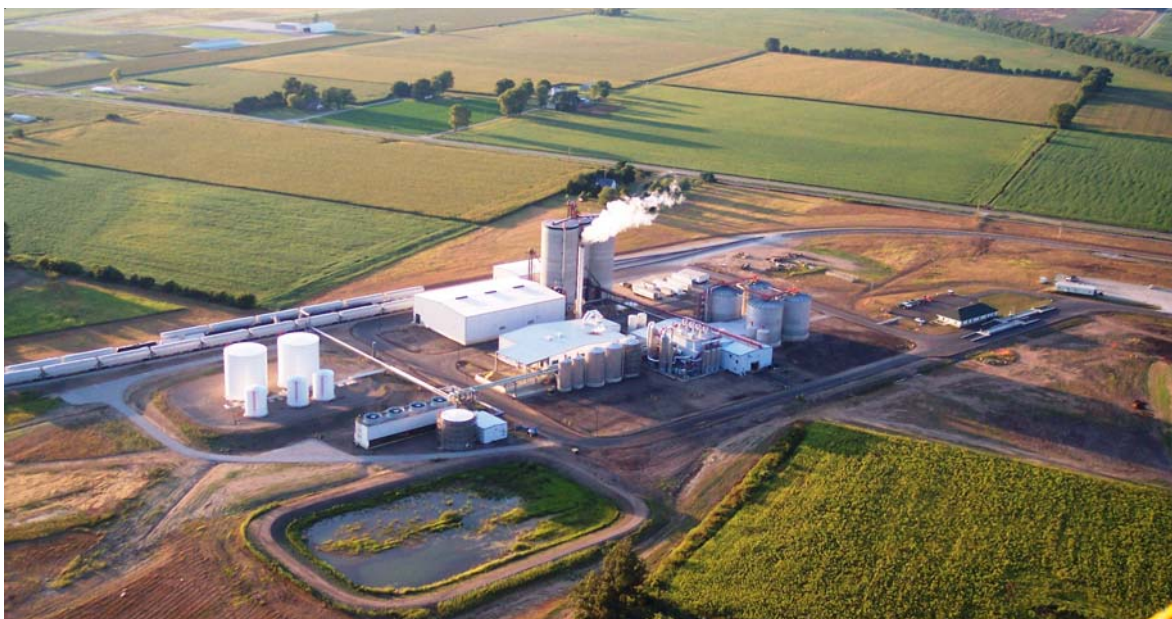
Figure 4: Aerial View of a Typical Ethanol Facility.
