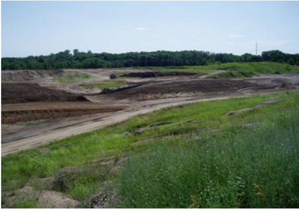
stabilization in the area before disturbing the next portion of the overall site. Soil exposure time is decreased, soil and erosion control practices are more manageable, and permit violations can be easily avoided.
