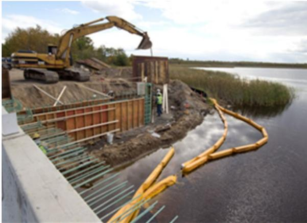
Use floating silt curtain for work in the water as secondary containment to contain sediment close to the work area.
