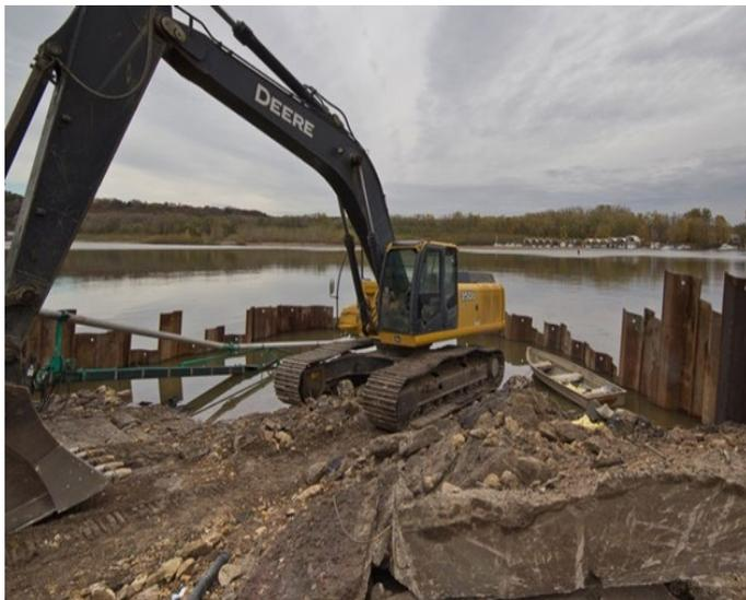
**Coffer dams made of sheet metal to isolate the work area from the surface water.**
