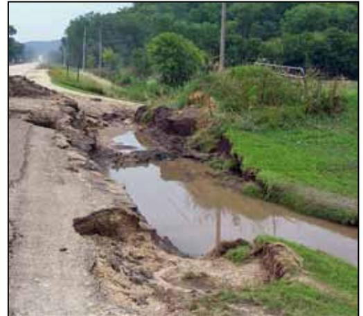
**A road near Elba, Minnesota, was damaged by flashfloods in August 2007.**
