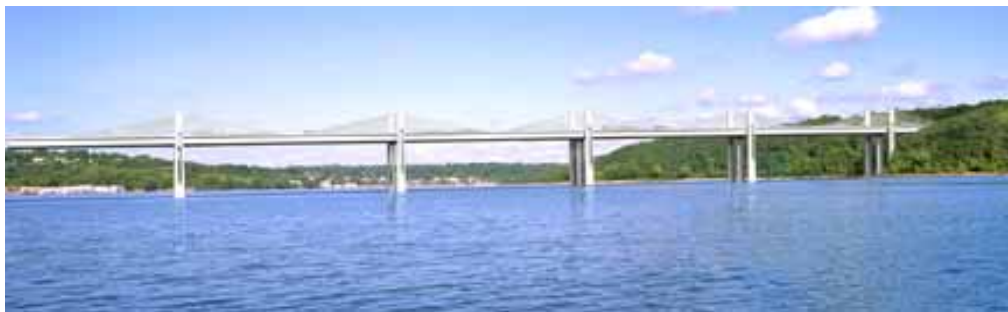
The proposed Stillwater Crossing (Courtesy Minnesota Department of Transportation)
