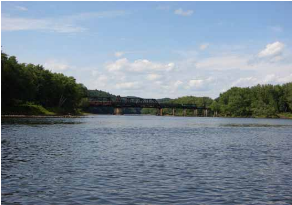
St. Croix River historic swing bridge near Cedar Bend (Photo by R.Ferrin)
