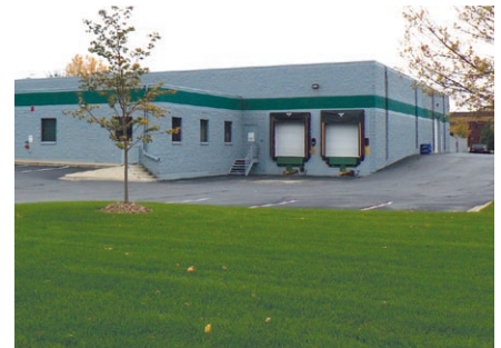
This industrial facility meets No Exposure requirements because materials and activities are kept indoors.
