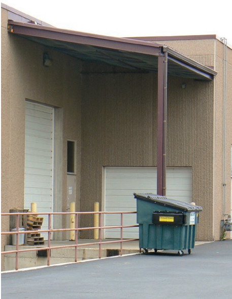
A closed dumpster and an awning over the loading dock keep significant materials from being exposed to stormwater.
