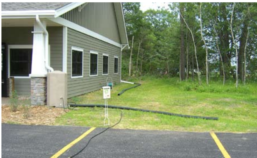
Fairview Office Park utilizes many LID techniques such as rain barrels, pervious asphalt and low-mow grasses
