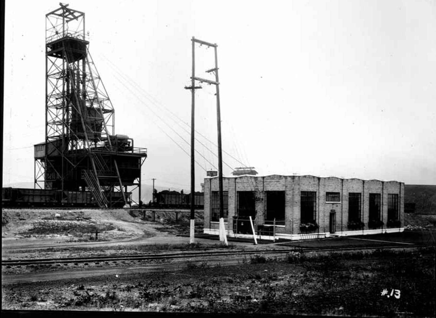
HEADFRAME AND HOIST HOUSE
