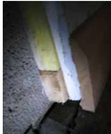
Remove ventilation diffuser
