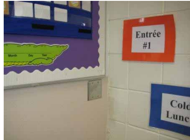
Cover with electrical plate when done
