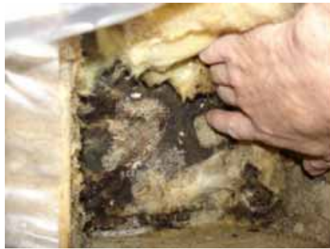
Pull away insulation
