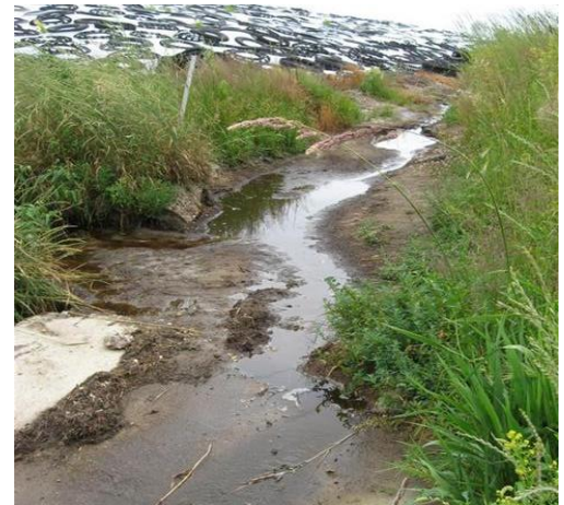
Leachate Being Generated
